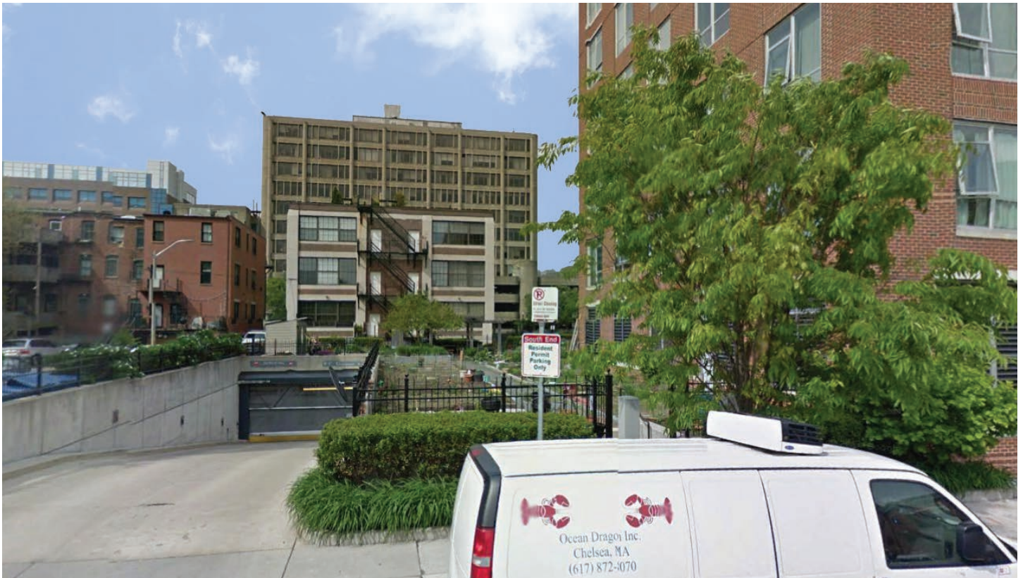
5 - East Canton Street Looking Southwest
