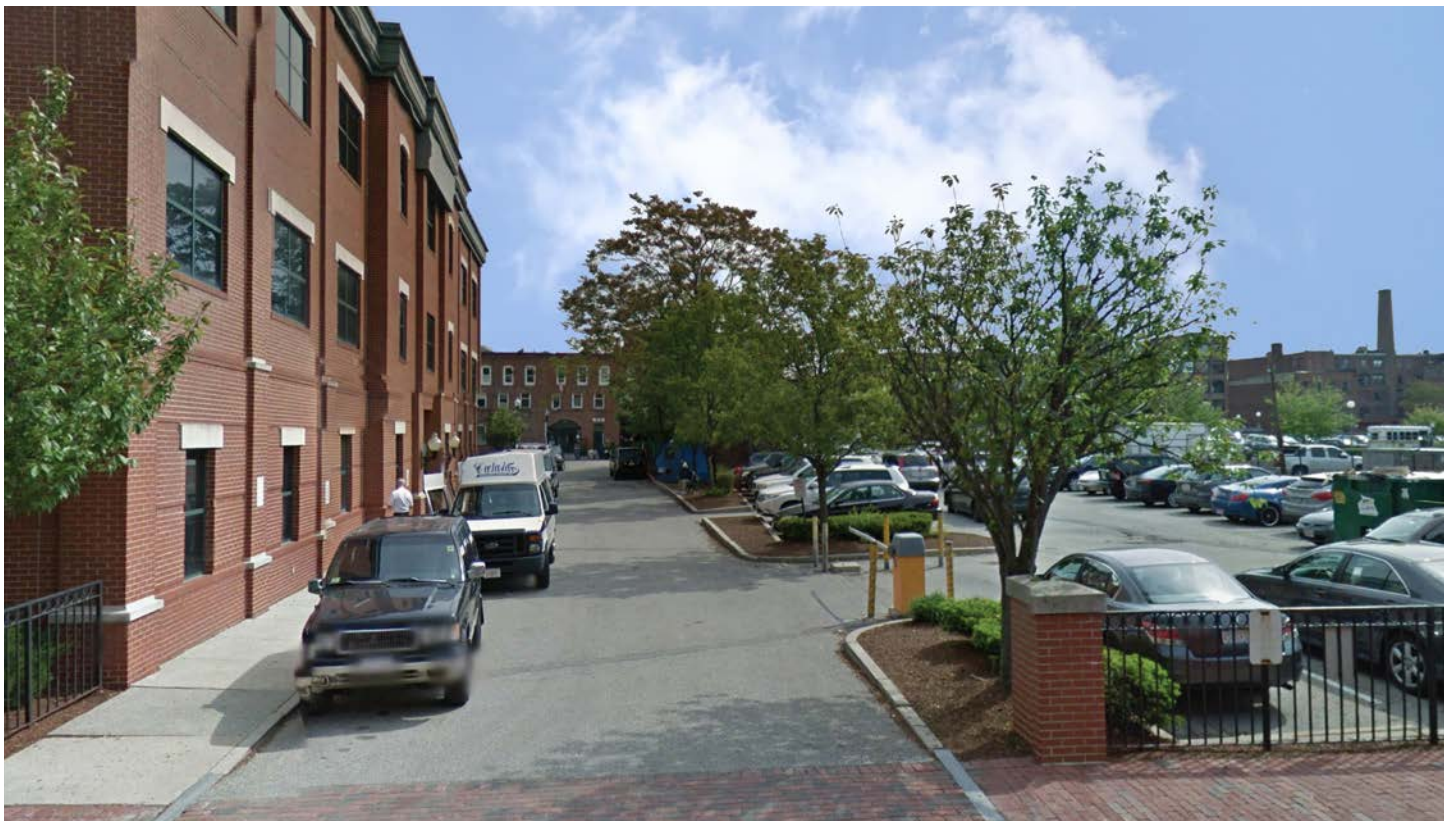
4 - Gambro Building at East Canton Street Looking Northeast
