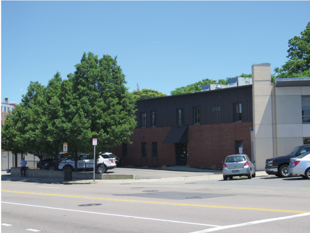
Figure 1-3. Existing Site Photos
