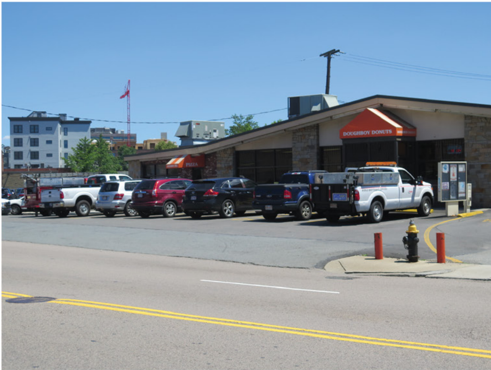
Figure 1-4. Existing Site Photos
