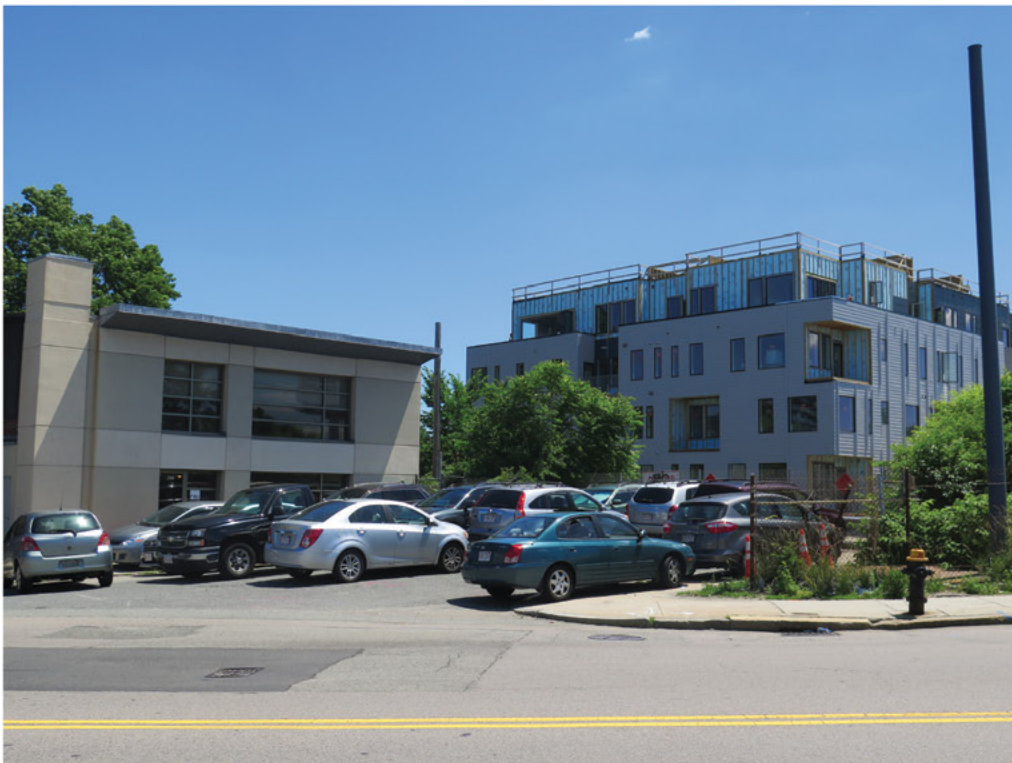
Parking on Private Street Next to Existing Building and Adjacent Residential Structure (Under construction) on Otherside of the Haul Road
