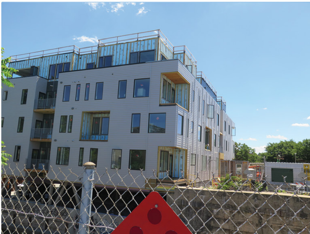
Rear New Building Under Construction Along Haul Road
