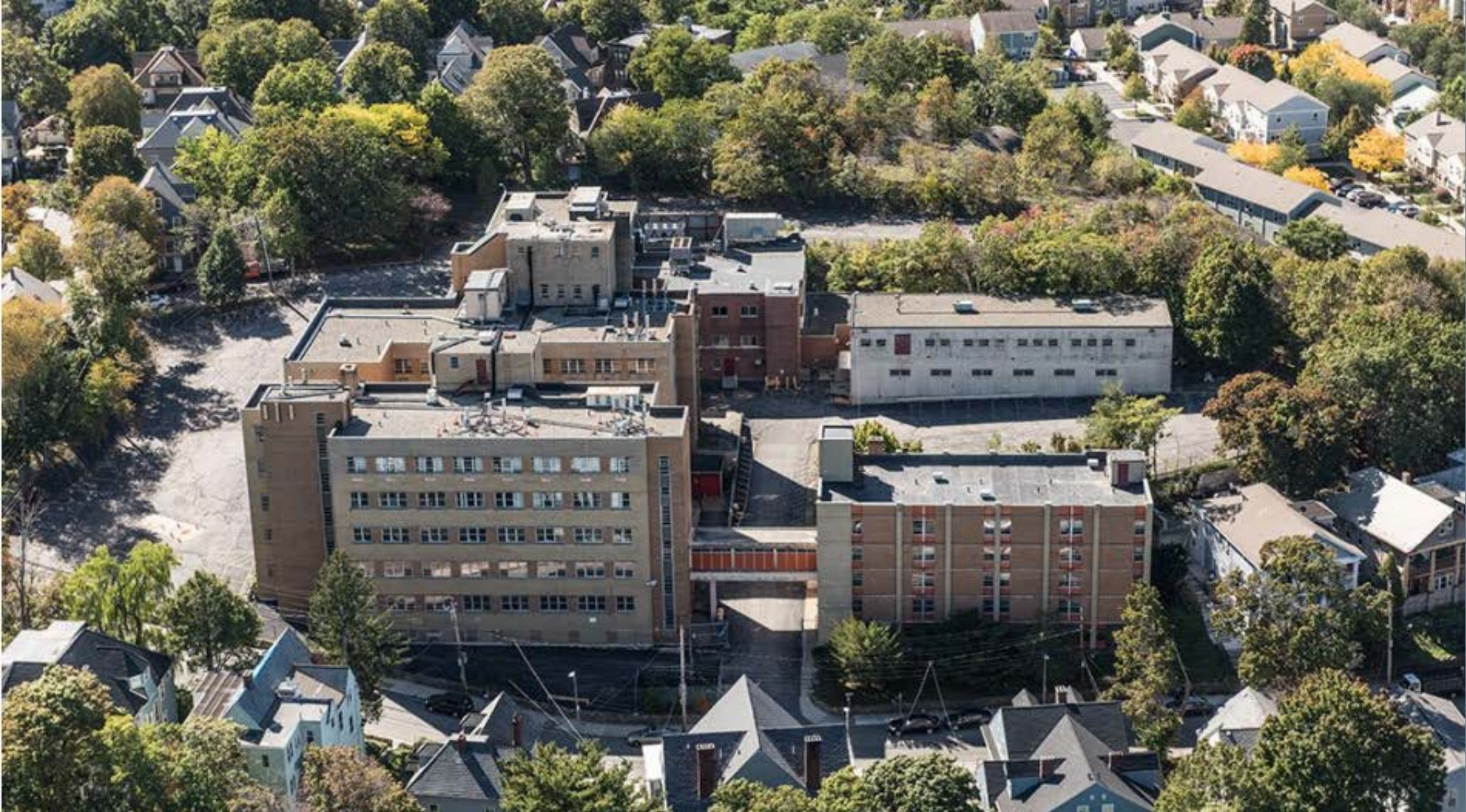
Existing Aerial View
