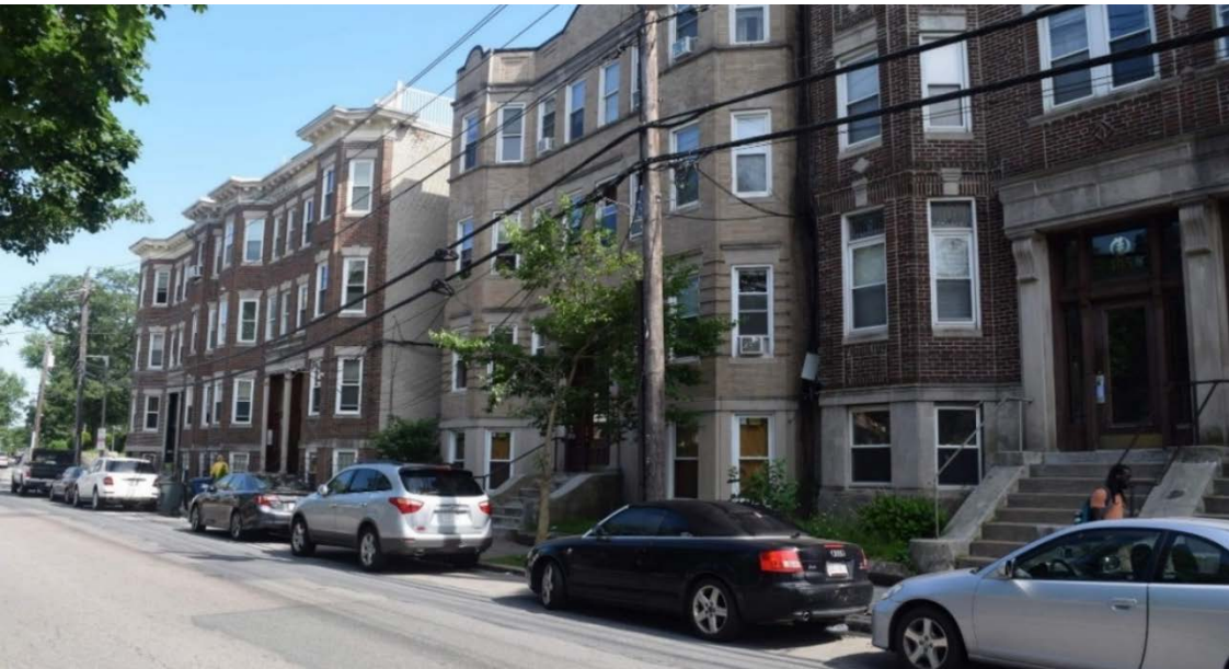
Apartments on Townsend Street across from Horatio Harris Park
