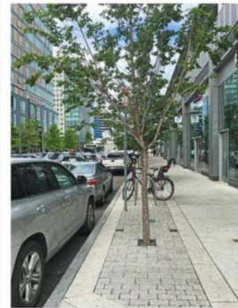
PRECEDENT IMAGE: GREENSCAPE + FURNISHING ZONE WITH PERMEABLE UNIT PAVING OVER STRUCTURAL SOIL
