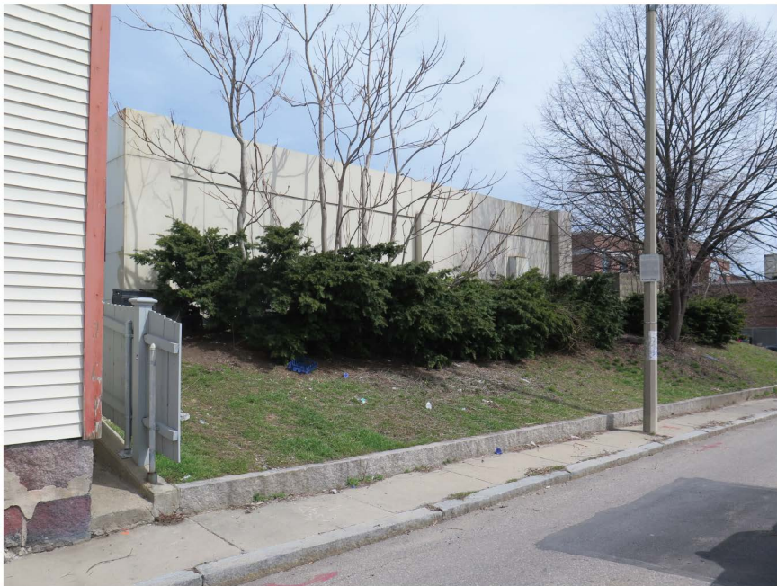
Rear of Existing Gas Station Along Silver Street
