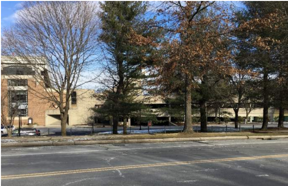
3. Beacon St Parking Garage
