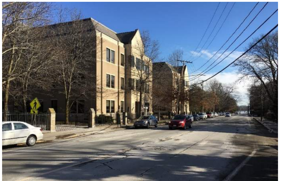
4. Merkert Chemistry Center (3 stories) – 36' from Beacon St
