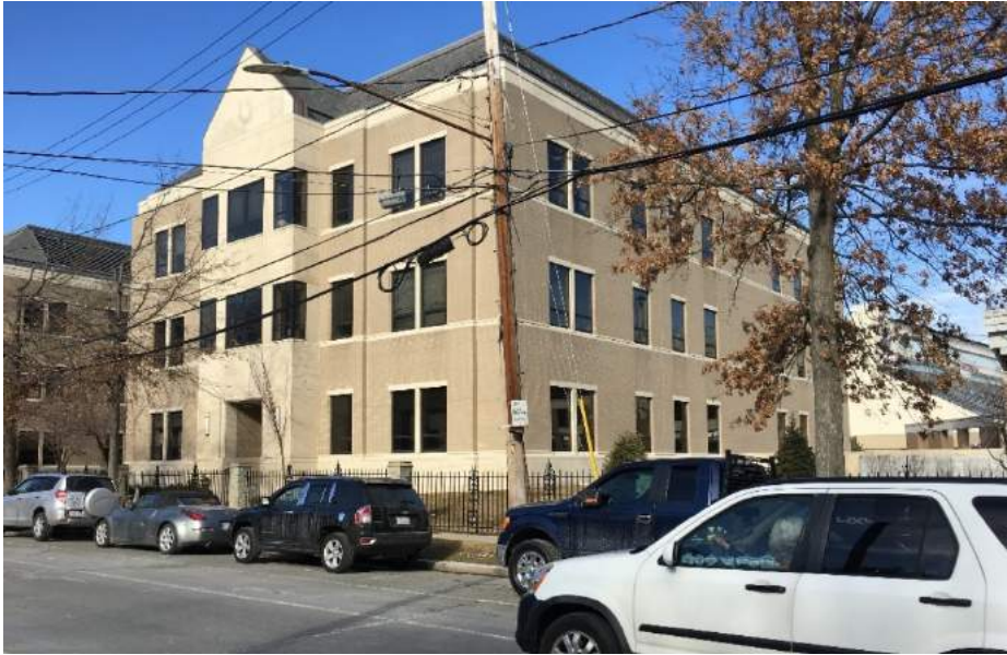
1. Merkert Chemistry Center (3 stories) – 36' from Beacon St
