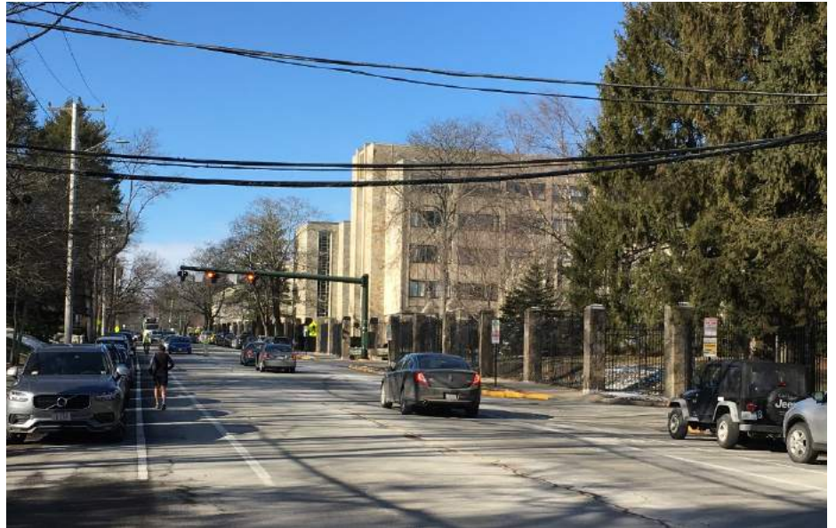
2. McGuinn Hall (5 stories) – 50' from Beacon St
