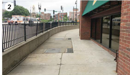
2 Existing site wall holding back grade along North Street.
