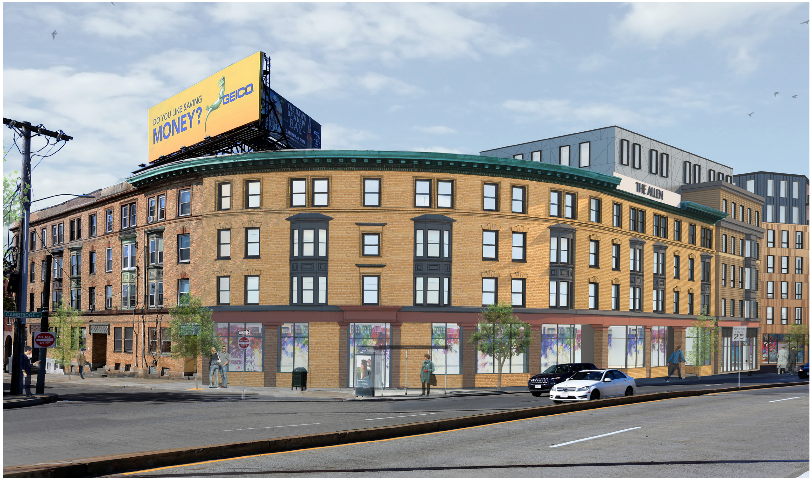
334 CAMBRIDGE ST (ALLEN BUILDING) - VIEW FROM CAMBRIDGE ST | EMBARC
