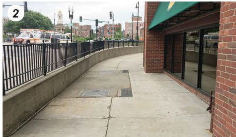
Existing site wall holding back grade along North Street.
