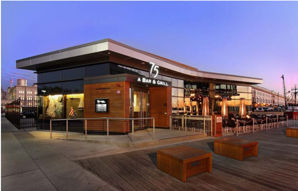
75 Liberty Wharf, Boston, MA CREDIT: PATRICK AHEARN ARCHITECT LLC
