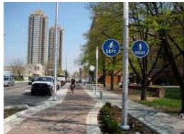
Special paving separates the at-grade bike path from the sidewalk, improving safety for walkers and bikers.
