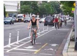
Two-lane cycle tracks offer protection from moving traffic.
