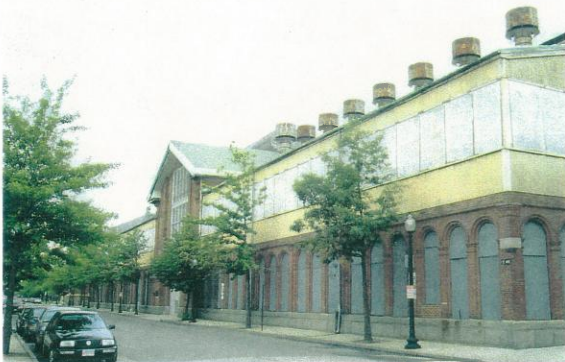
View looking to the west showing the principal elevation on First Avenue.
