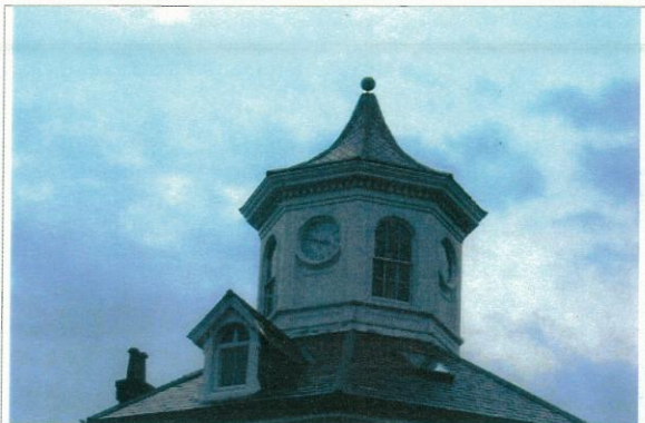
View looking west at upper portion of roof.
