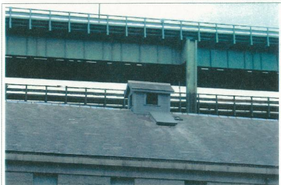
View looking west at stabilized cupola and covered skylight.
