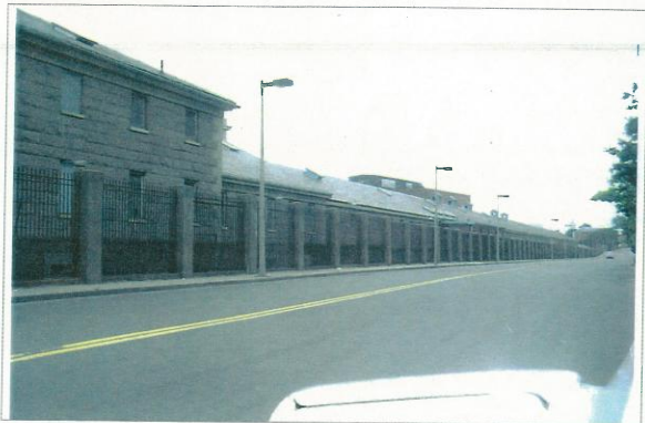
View looking south showing northwest elevation of Ropewalk along Chelsea Street.
