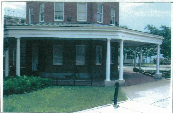
Detail view looking east showing restored canopy and ground plane.
