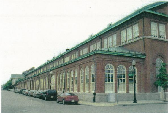
View looking west along First Avenue from Sixteenth Street.
