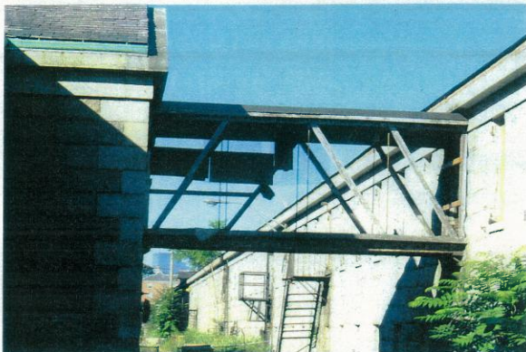
Looking southwest at stabilized bridge between Ropewalk and Tar House.
