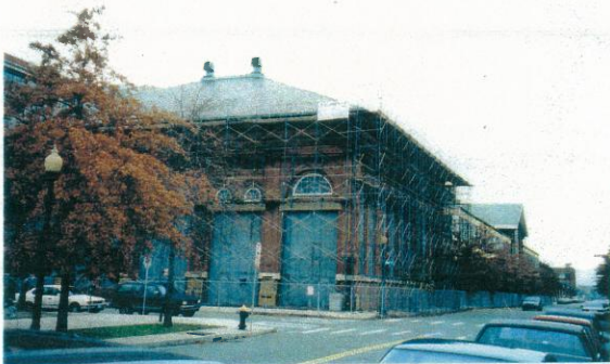
General view looking north along First Avenue showing project nearing completion.
