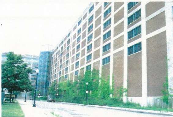
Oblique view looking west showing southeast elevation and elevator tower at west end.
