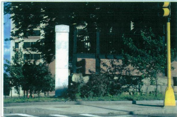
Detail view of west side of Gate 6 showing new granite post and restored brick and stone wall with iron fence. 7/23/00
