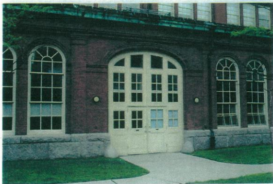
Typical side entry detail of northwest elevation from Second Avenue.
