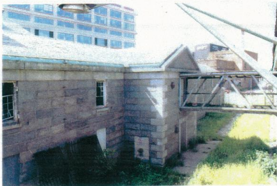
Looking south from the Ropewalk at the Tar House before stabilization.
