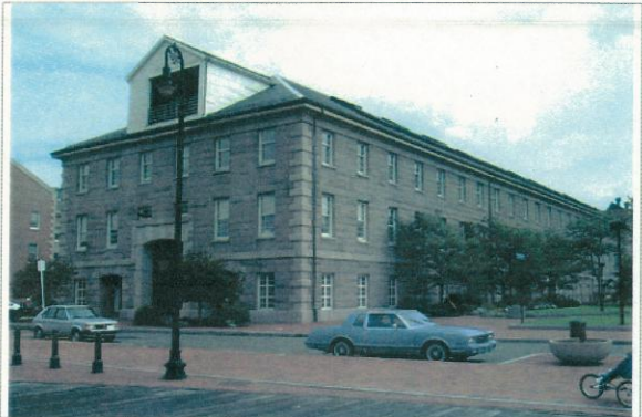
View looking North Across Sixth Street
