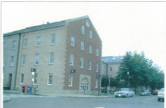
View looking north showing southeast and southwest elevations.
