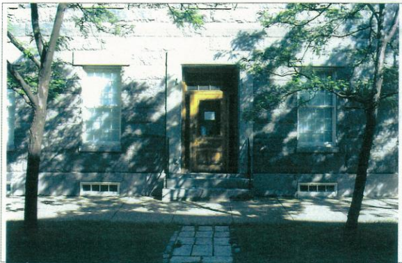
Looking northwest at typical side entrance facing Second Avenue.
