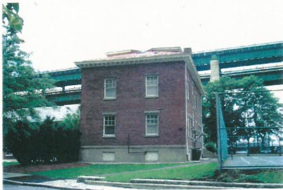
View looking northwest showing southeast elevation.
