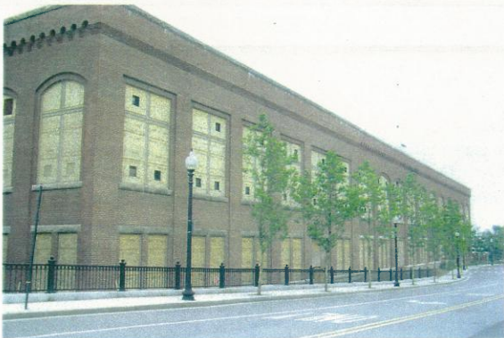
View looking east showing southwest elevation and Sixteenth Street access to Gate #6.
