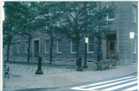
View looking west showing restored stairs, doors, windows and basement sash on southeast elevation facing Second Avenue.
