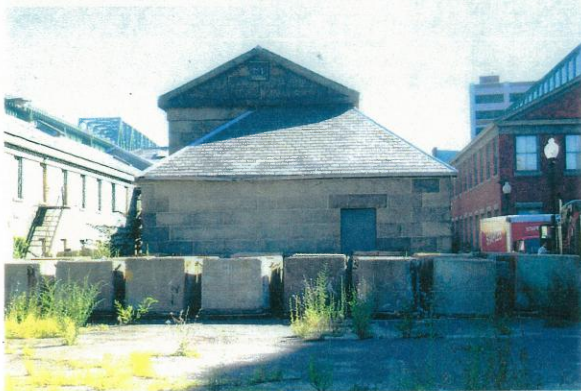
Looking north at the Tar House addition which required nearly 100% repointing.
