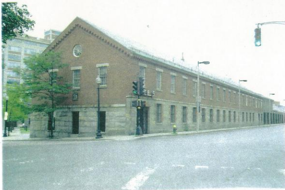
View looking to the southwest along Chelsea Street showing the northwest elevation of Building 79.
