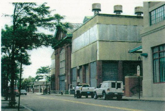
View looking south at Thirteenth Street elevation showing encapsulation at windows for HazMat mitigation.
