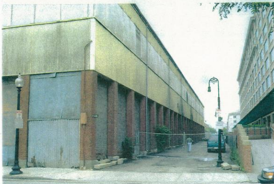
View looking southwest along Second Avenue at northwest elevation.
