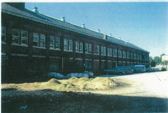
View looking southwest at northeast elevation. Note restored gutter and roofing.
