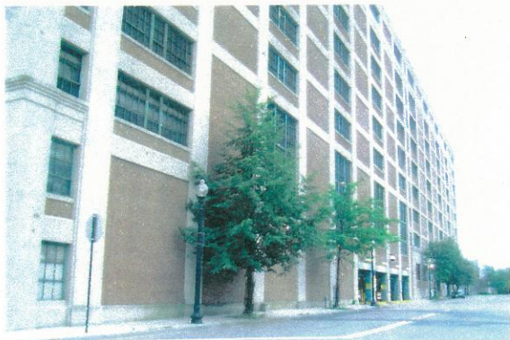
Oblique view of northwest elevation.
