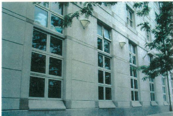
Detail view at first floor level showing building details.
