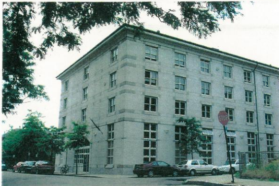
Detail view looking south showing northeast elevation and part of northwest elevation.
