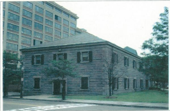
View looking south from Thirteenth Street near Gate 5 showing original portion of building. 6/29/00
