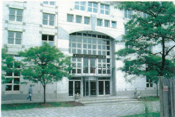
View looking northwest across Second Avenue at main entrance to Building 150.
