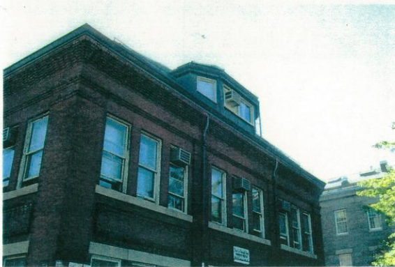
Detail of southwest elevation showing restored dormer, gutter and downspouts.
