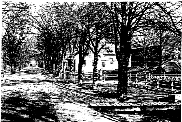
Main (Second) Avenue, looking east.
