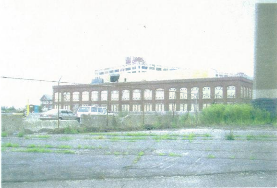
View looking southwest from Moran Terminal showing northeast elevation of Building 114.
