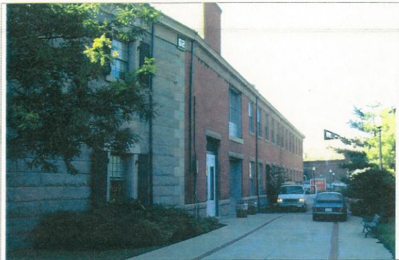
View looking southwest showing northwest elevation showing later brick addition.
