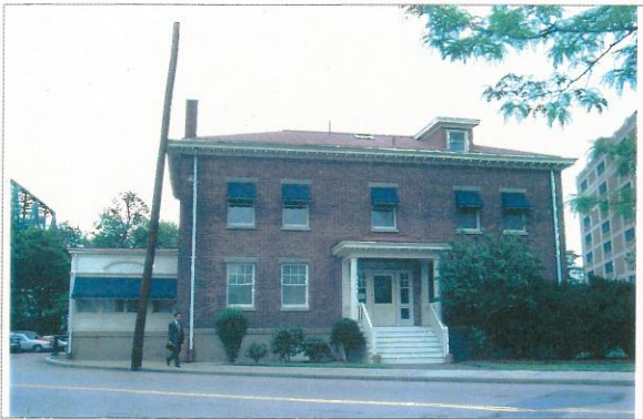
View looking northeast at front elevation on Thirteenth Street.
