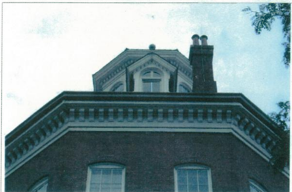
View showing detail of upper cornices.
