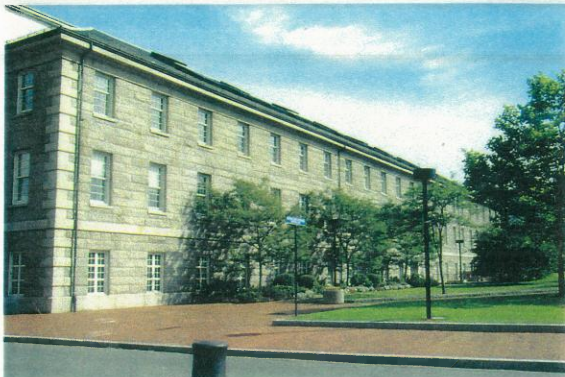
View looking north at southeast elevation of the building.
