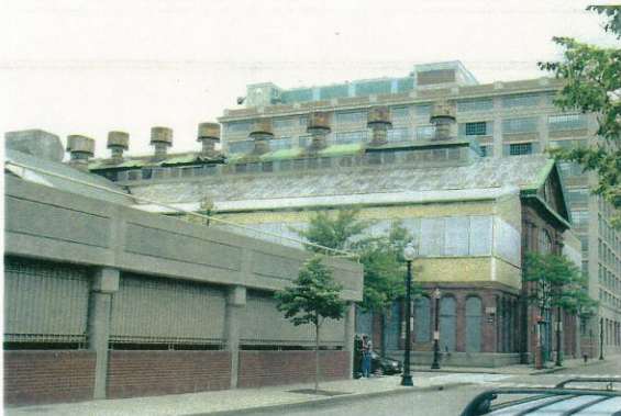
View looking west at the northeast end of the building at First Avenue and Thirteenth Street. 6/29/00
