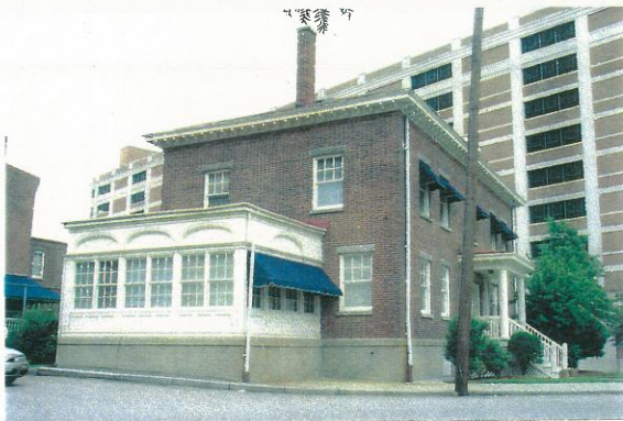
View looking southeast showing northwest elevation.
