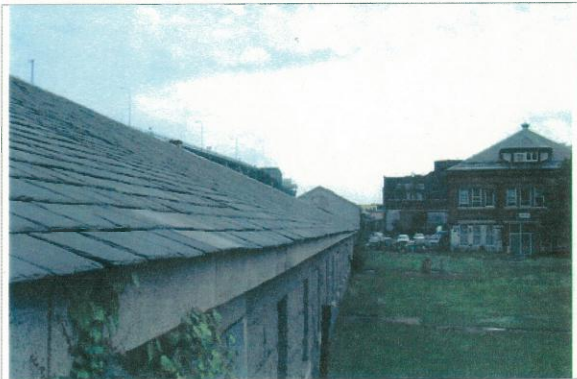
View looking northeast along cornice line of southeast elevation.
