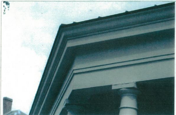
View of detail of porch cornice.
