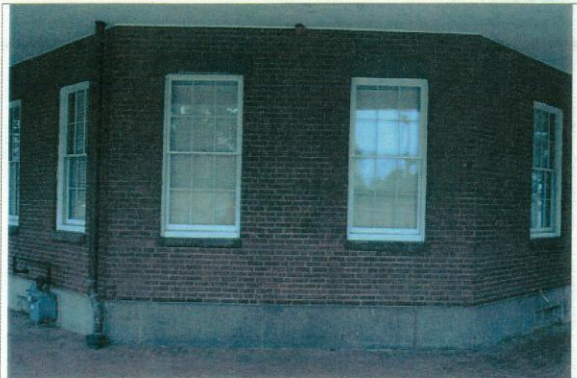
Detail view looking northeast showing first floor elevation.
