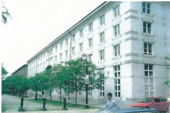
View to the west showing the front elevation facing Second Avenue.
