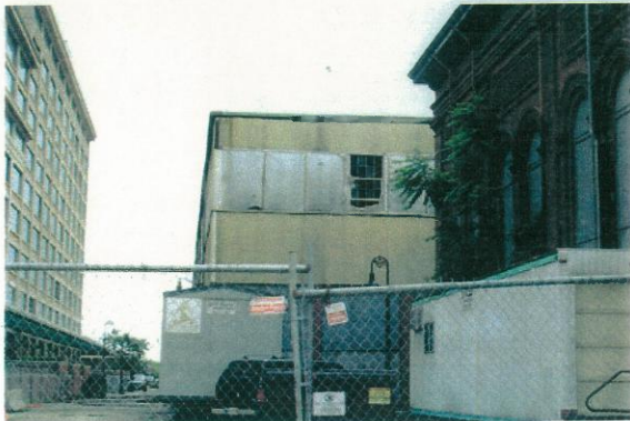
View looking northeast showing stabilization repairs and encapsulation for HazMat mitigation. 6/29/00
