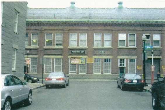
View looking northwest at the southeasterly side of building. Note historic signage.
