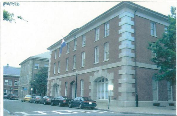
View looking north showing restored Seventh Street elevation.
