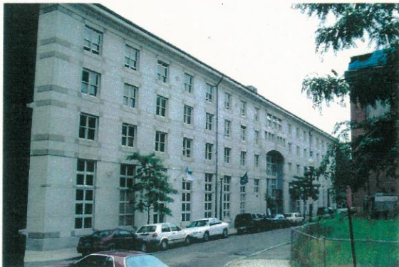
View looking south showing northwest elevation along Third Avenue.
