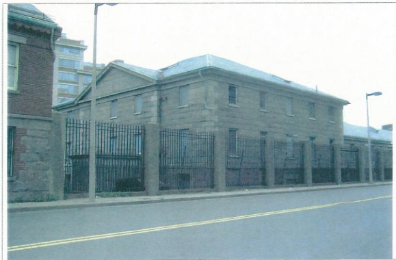
View looking south across Chelsea Street at Ropewalk Headhouse.
