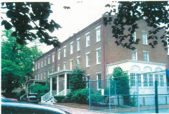
View looking northeast at front elevation .
