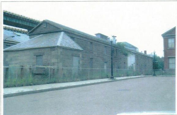
View to north from Fourth Avenue showing east elevation of Building 60. 7/16/00
