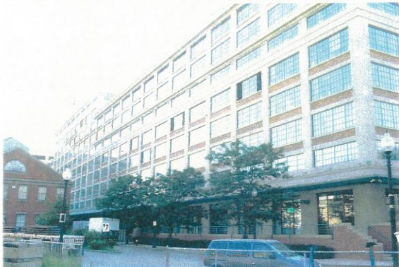
Looking east at oblique view of northwest elevation.
