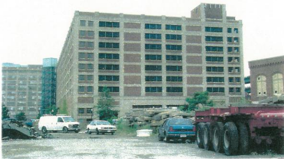
View looking southwest at northeast elevation.
