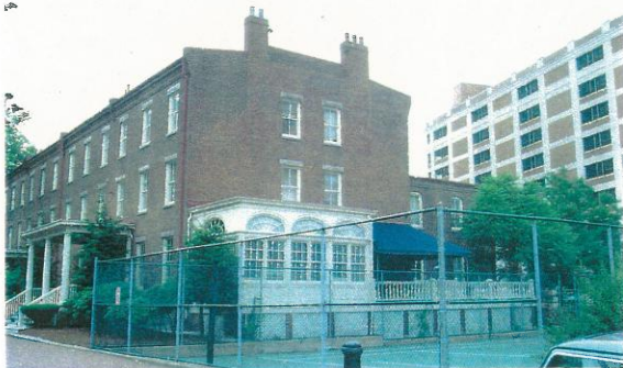
View looking northeast showing southwest elevation.
