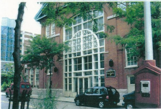
Detail view of entrance on Thirteenth Street.
