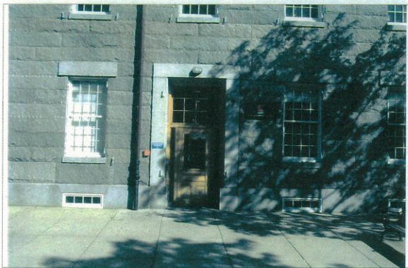
Looking northwest at main entrance facing Second Avenue.
