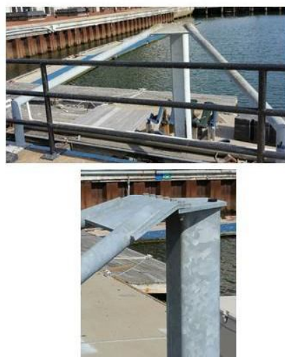
Metal Piles Anchored to Granite Dry Dock Wall
