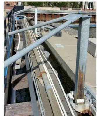
Metal Piles Anchored to Granite Dry Dock Wall
