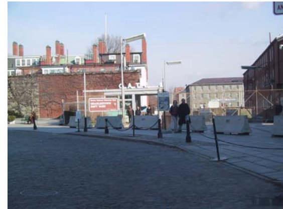
Gate 1 is a major entrance to the Navy Yard for visitors on the Freedom Trail and for Charlestown residents. The chain link fence, lack of signage with information about the entire Yard, and concrete barriers provide an unwelcoming environment.
