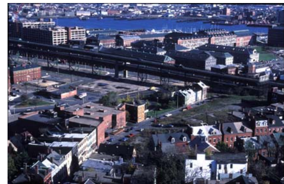
The Tobin Bridge overpass is one of many barriers to entry to the Navy Yard. The overpass, busy Chelsea Street with its few pedestrian crossings, and the brick wall around the Navy Yard all contribute to the Yard's character of a "gated community."
