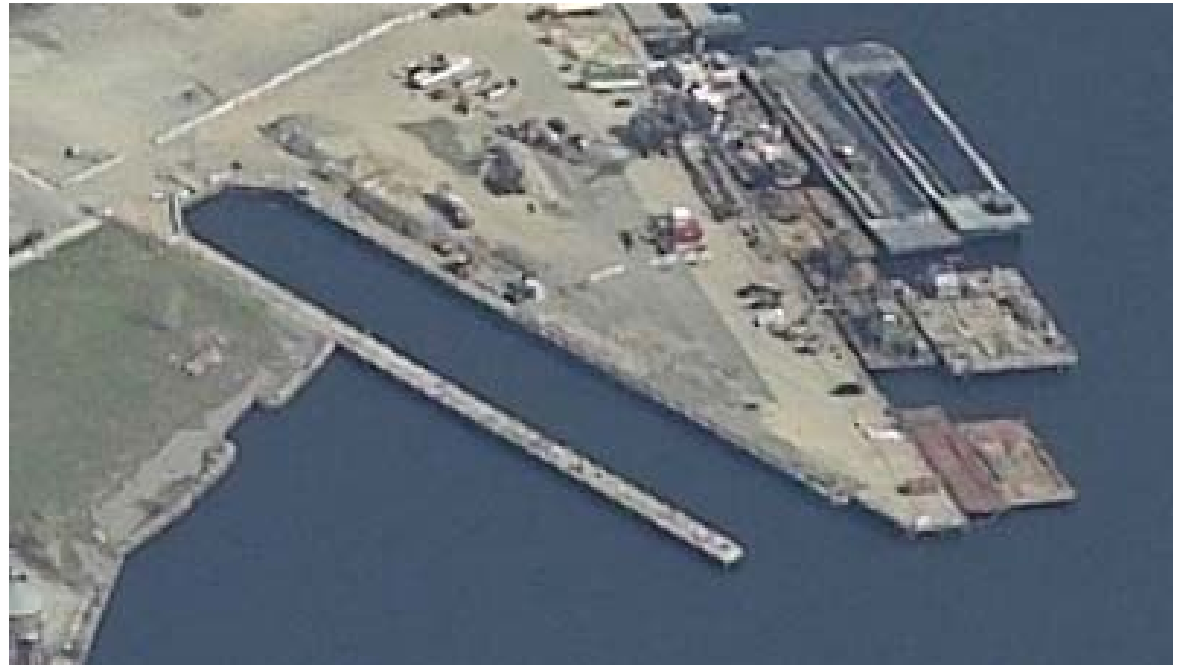
Dry Dock 5 currently exists as under-utilized space.
