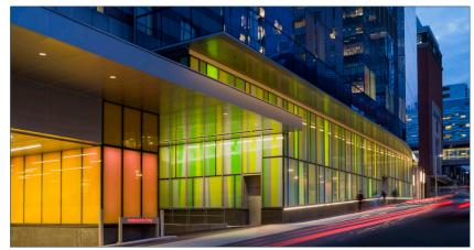
The Mandell Building's facade was lit in a sealed environment – no one would be able to get in for maintenance. Thus, fiber optics were used to ensure longevity of the system.
