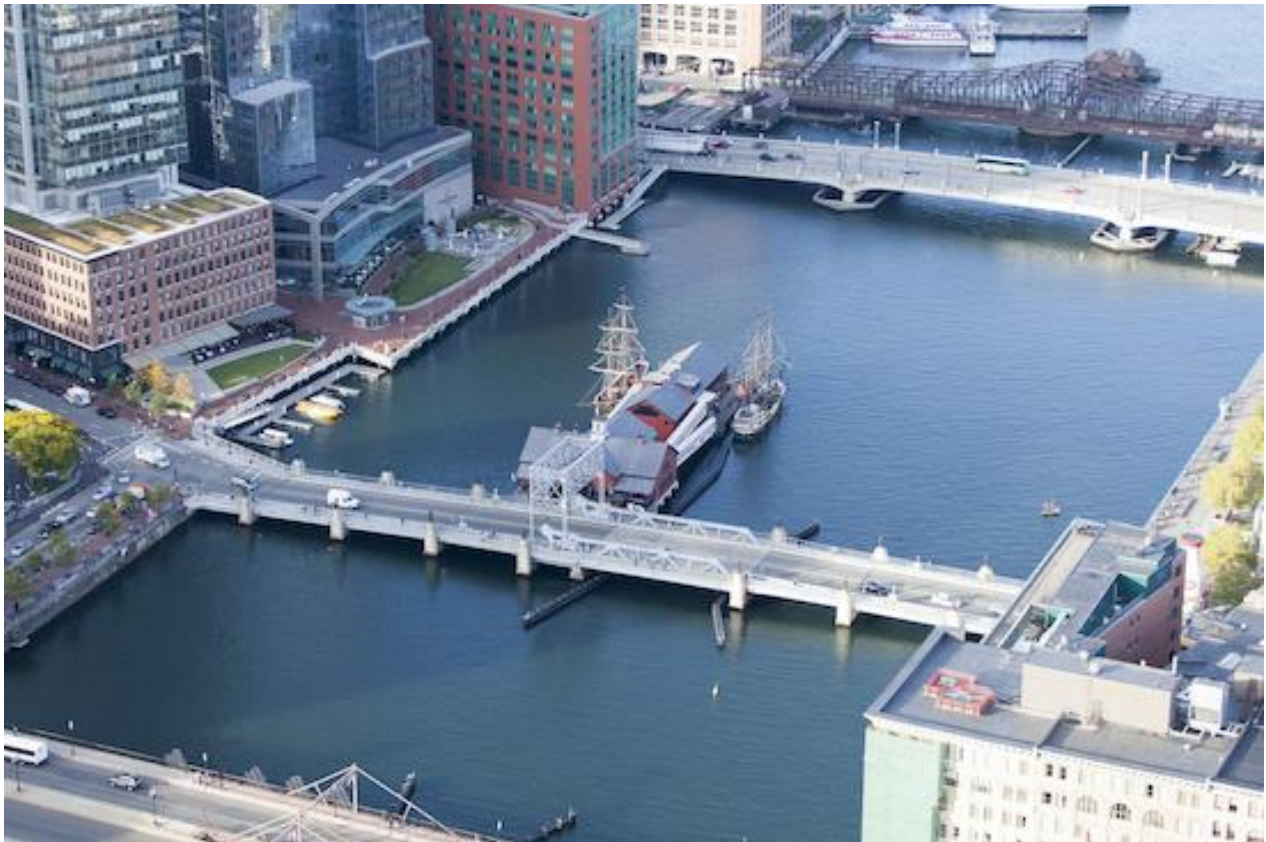
Site area: Fort Point Channel Congress Street Bridge
