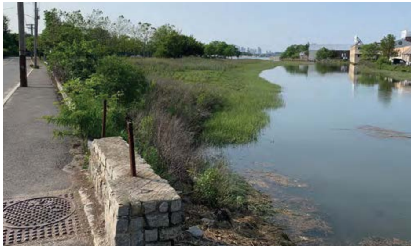
Figure 38: Pine Neck Creek outfall and existing marsh
