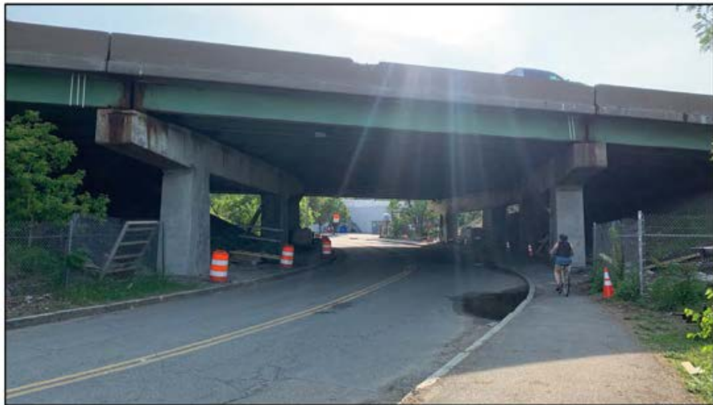
Photo 6: Inland-facing view of Conley Street as it passes through the Expressway underpass/location of the Conley Street flood pathway.
