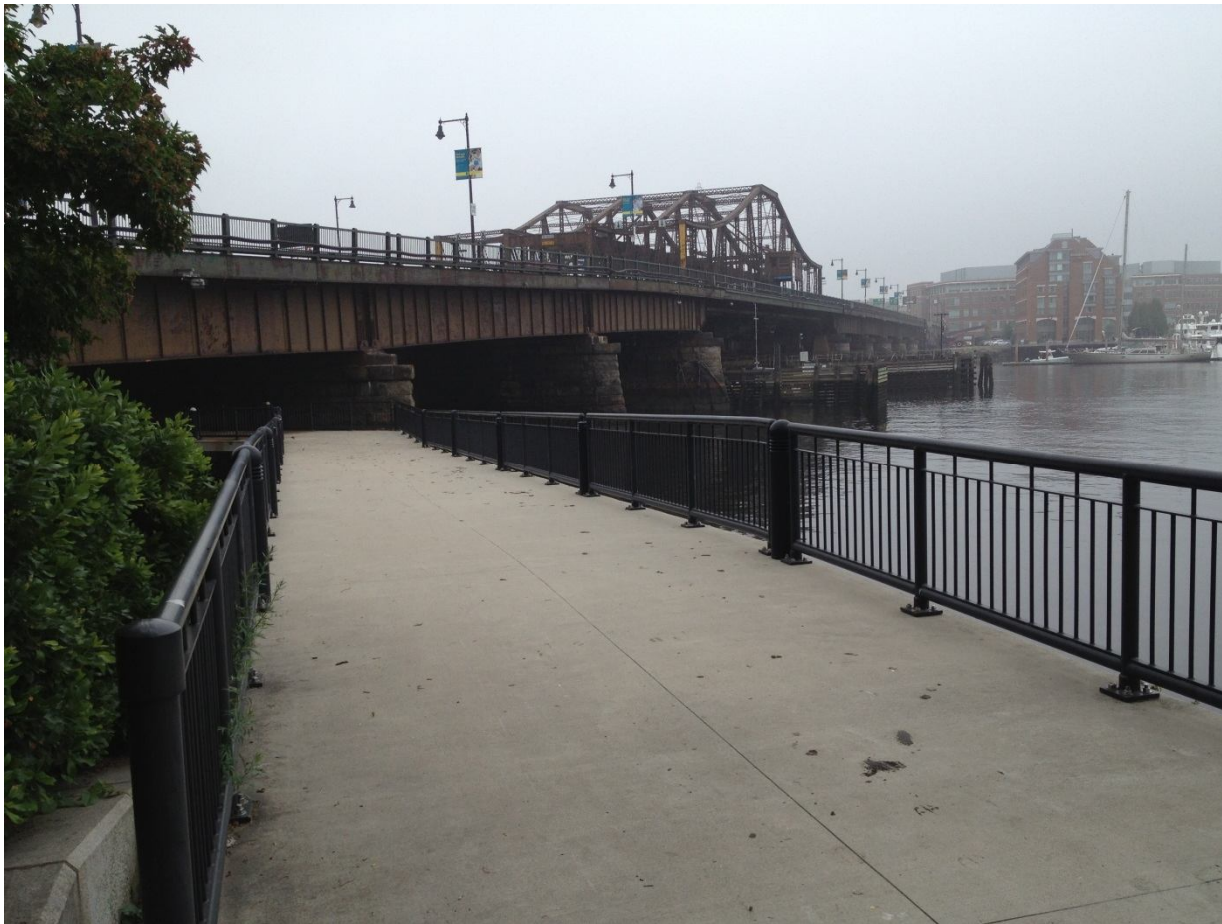
North Washington Street Bridge
