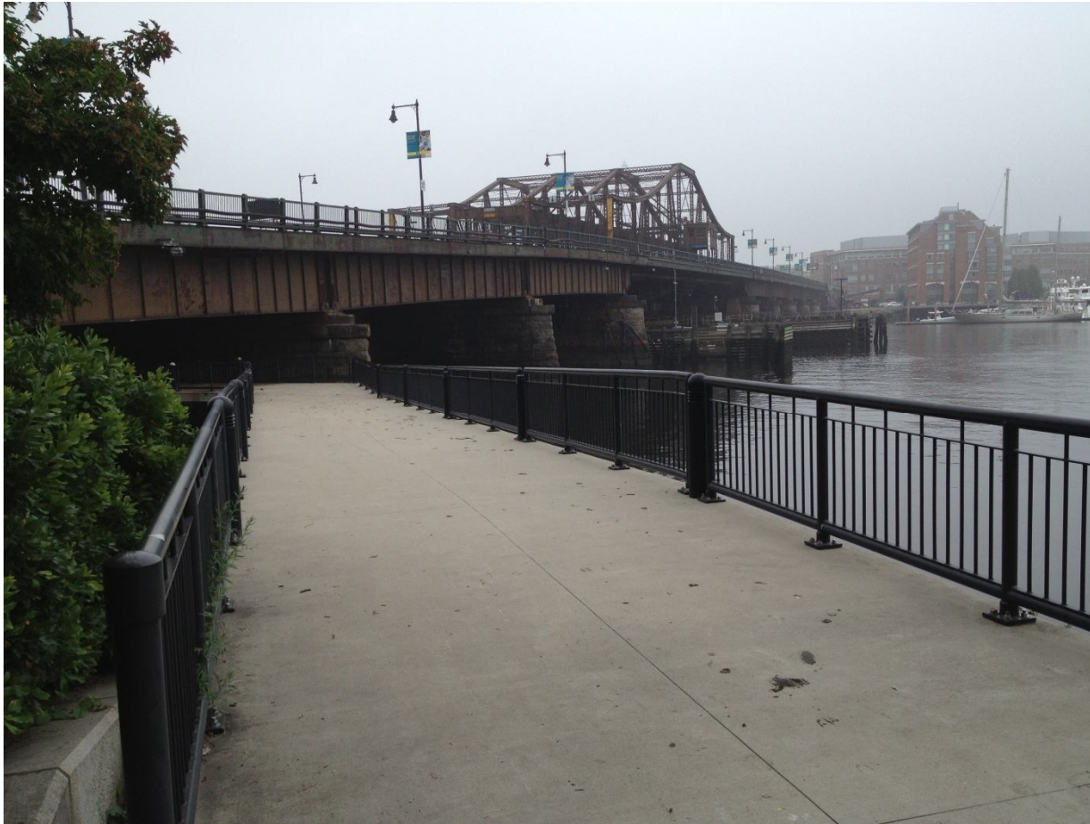
North Washington Street Bridge
