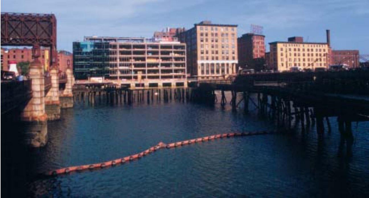
An abandoned water line between Congress Street and Summer Street will be removed as part of the Congress Street Bridge reconstruction. This improvement will enhance the overall identity of the waterway and open the way for productive use of this section of the Channel. A new Harborwalk segment at 303 Congress Street recently opened.
