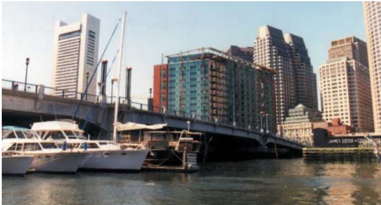
The 16-foot vertical clearance of the fixed Evelyn Moakley Bridge at Mean High Water (MHW) is the limiting factor for vessels seeking to enter the Channel.
