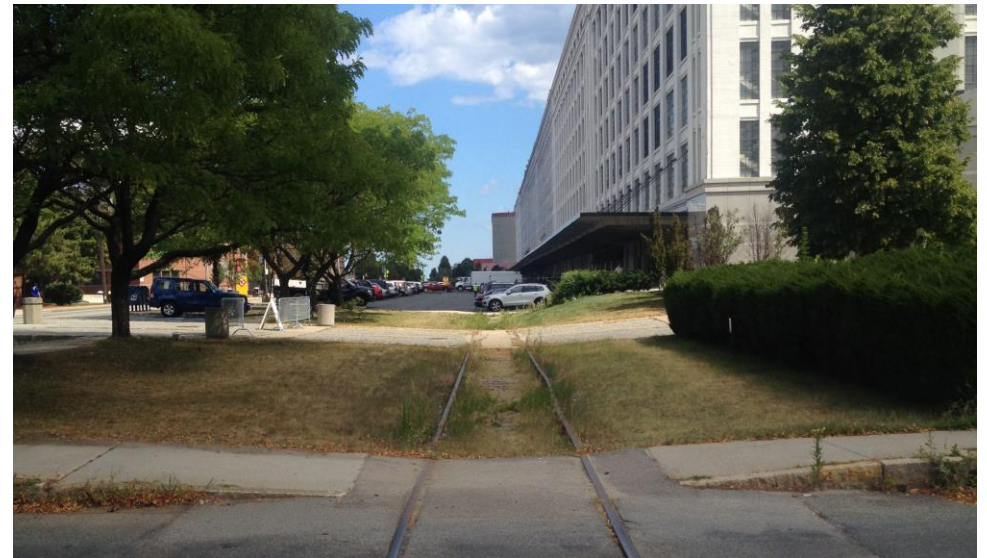
Challenges for reactivating Track 61 and repairing waterside infrastructure make cargo opportunities difficult.
