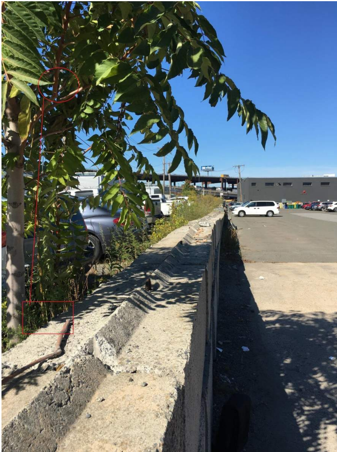
FIGURE 6: Side view at Location #3 microphone (oval) located off tree branch. Leaves around microphone to be removed. Instrumentation to be located on the opposite side of the concrete block on the ground.
