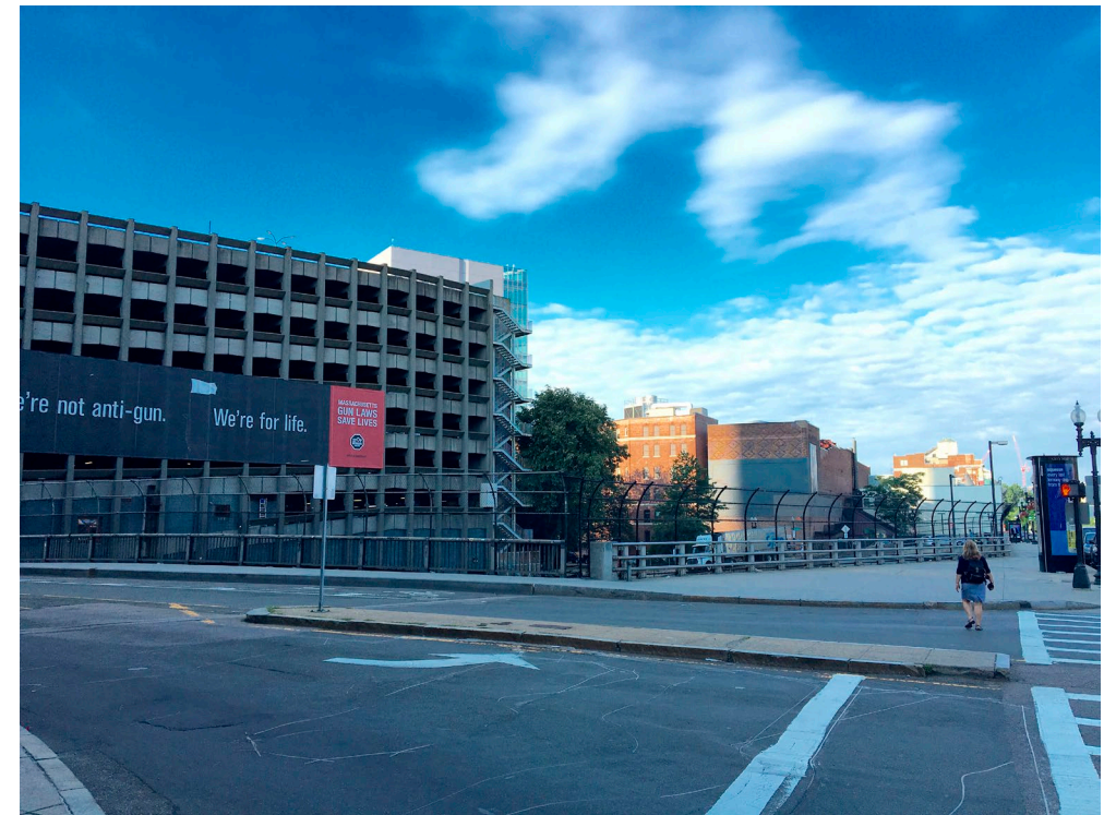
Corner of Dalton Street and Boylston Street looking West
