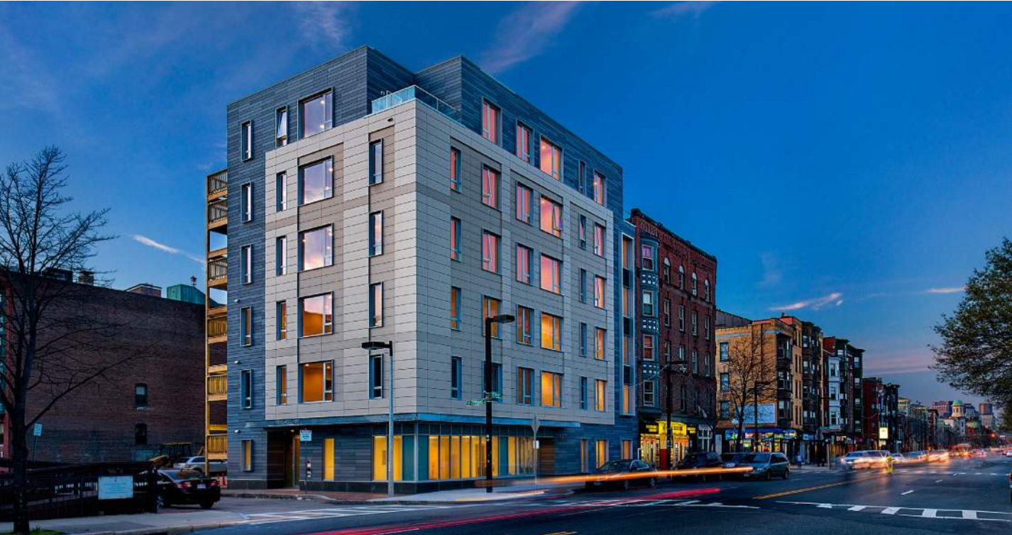
Completed Phase I South West
