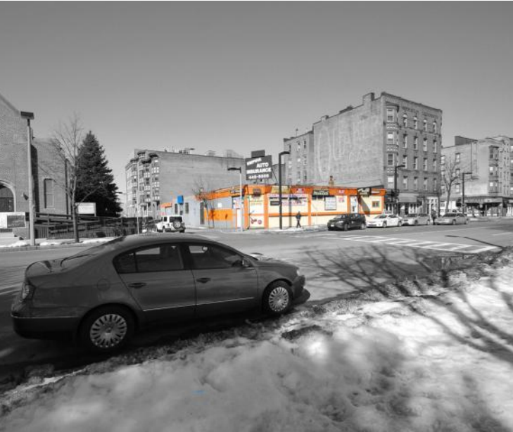
Existing Conditions from South West
