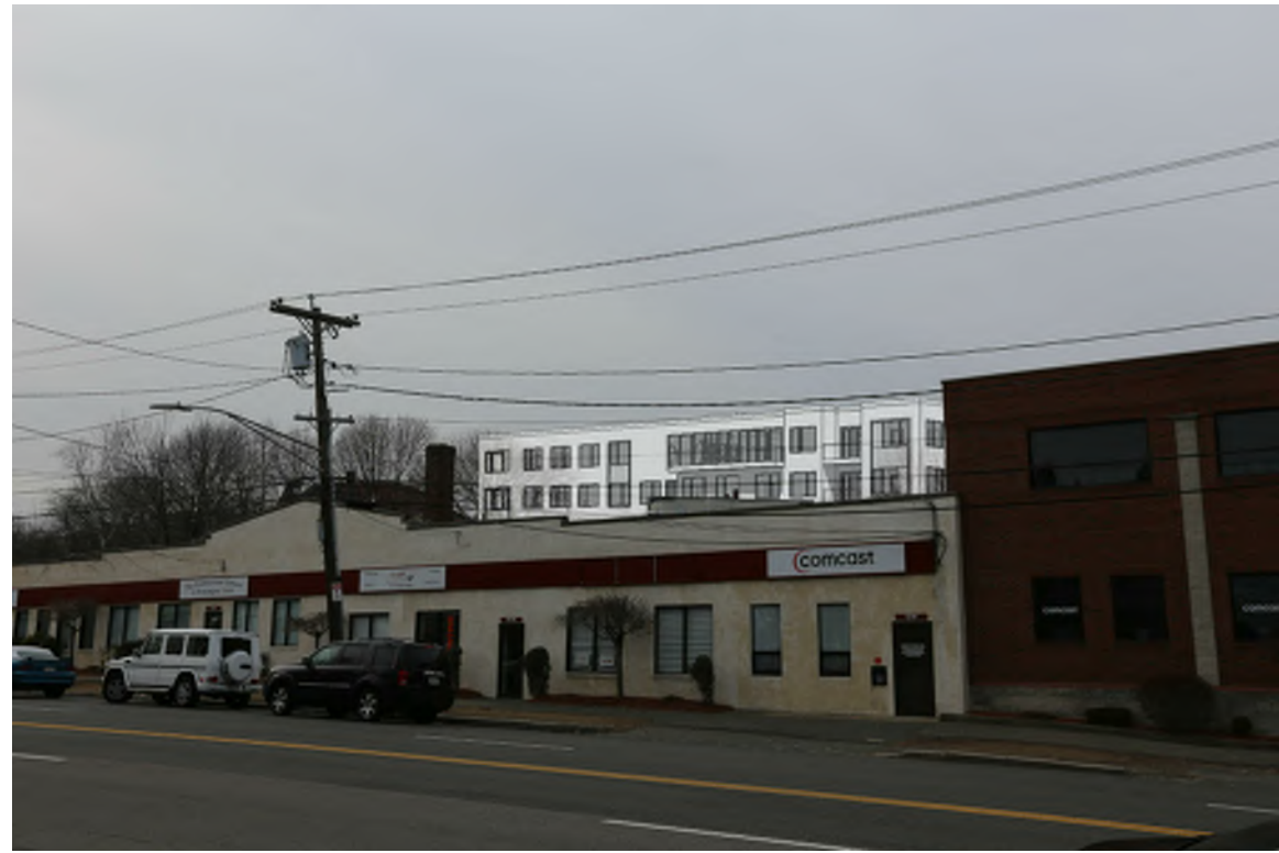
VIEW 2 LOOKING WEST ACROSS BENNINGTON STREET
