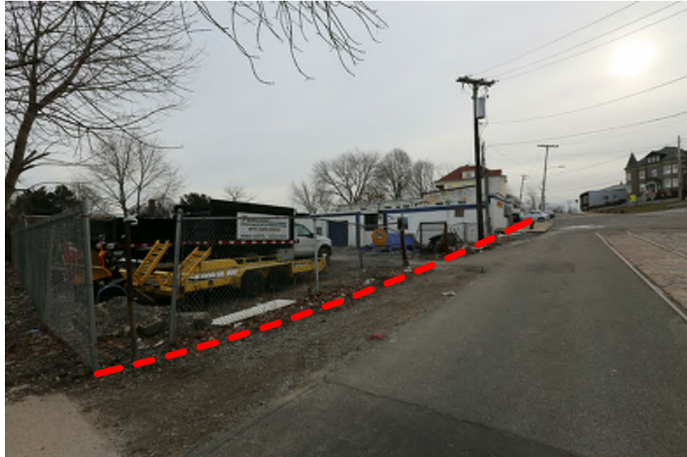
VIEW 2 NORTHWEST CORNER OF SITE FROM WALLEY STREET
