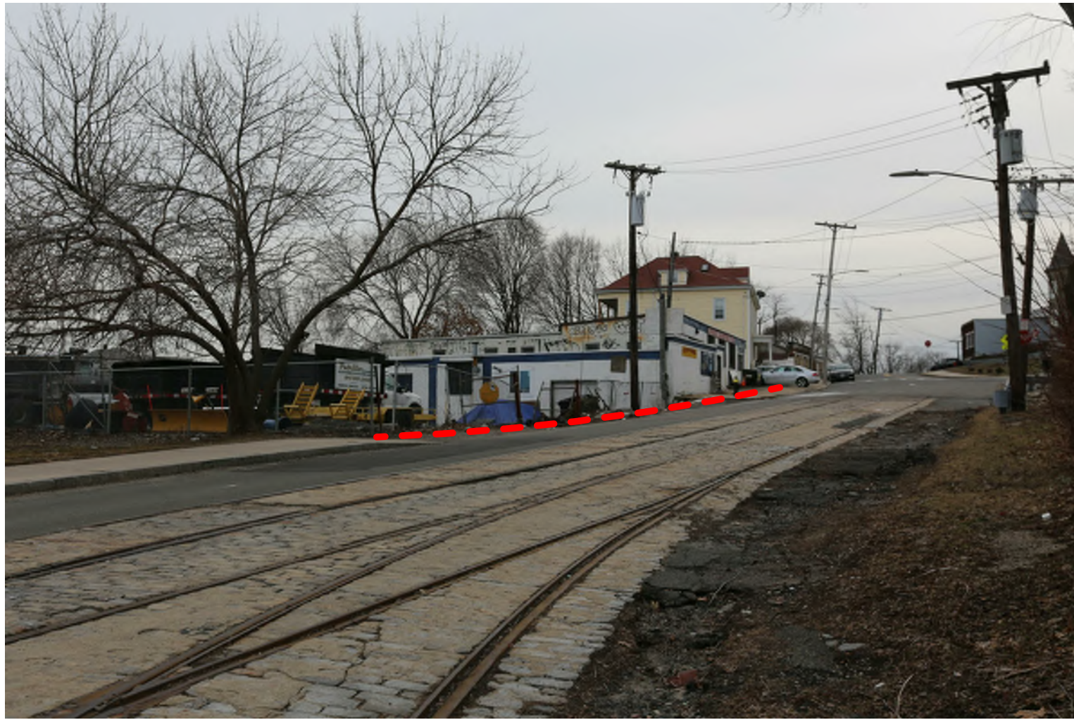
VIEW 1 LOOKING SOUTH UP WALLEY STREET
