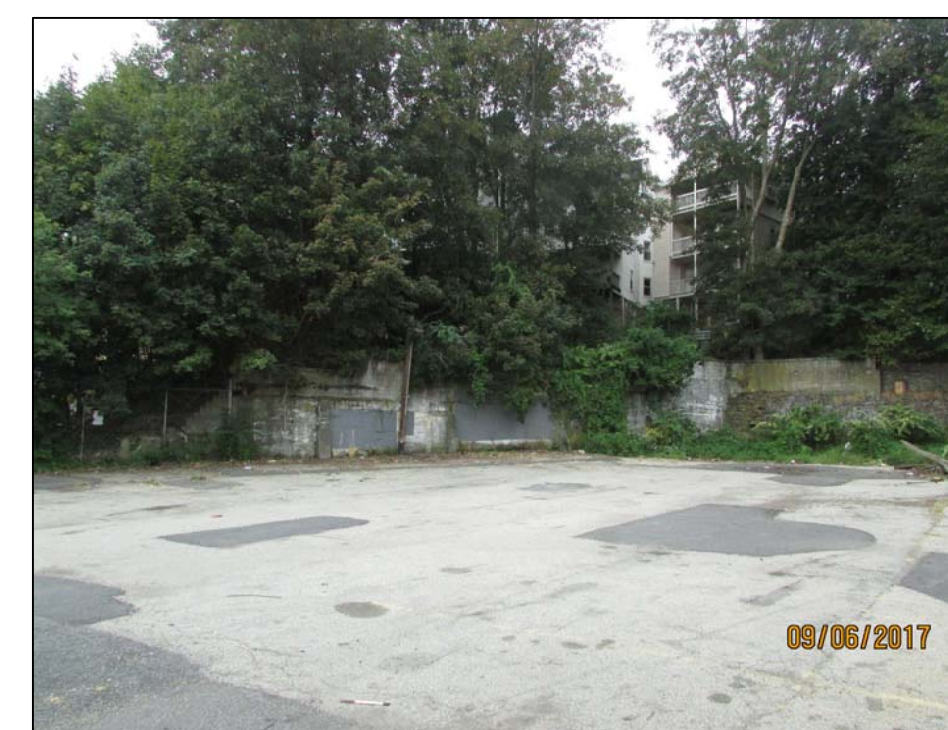
EXISTING REAR OF SITE / EXT. WALL
