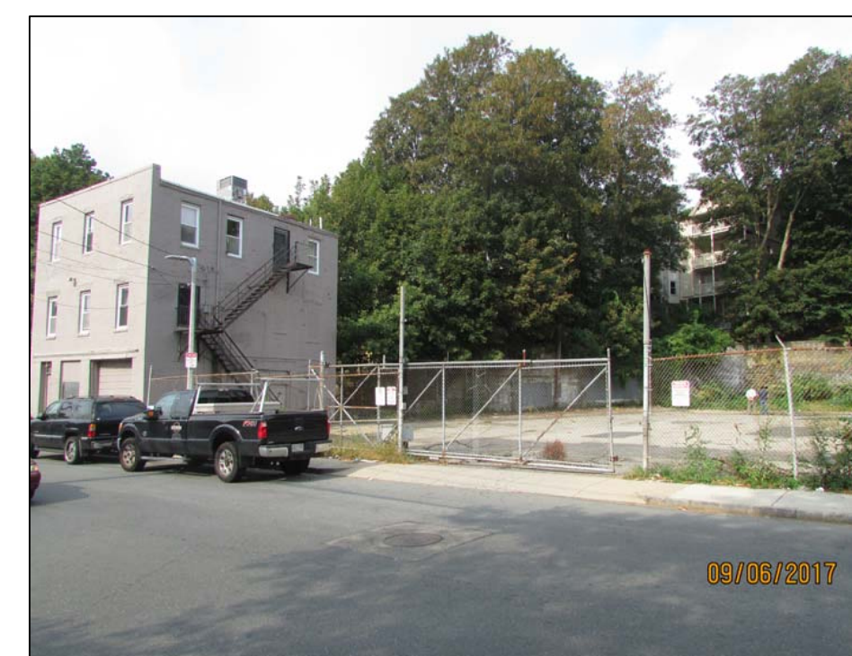
EXISTING BUILDING / EXISTING SITE
