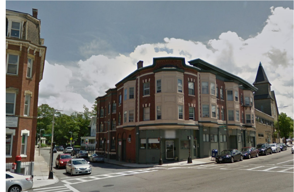
138-148 Warren St. at Moreland St.
