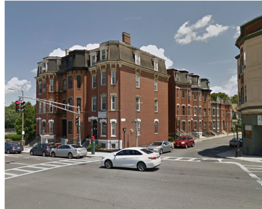
132-136 Warren St. at 2-6 Moreland St.
