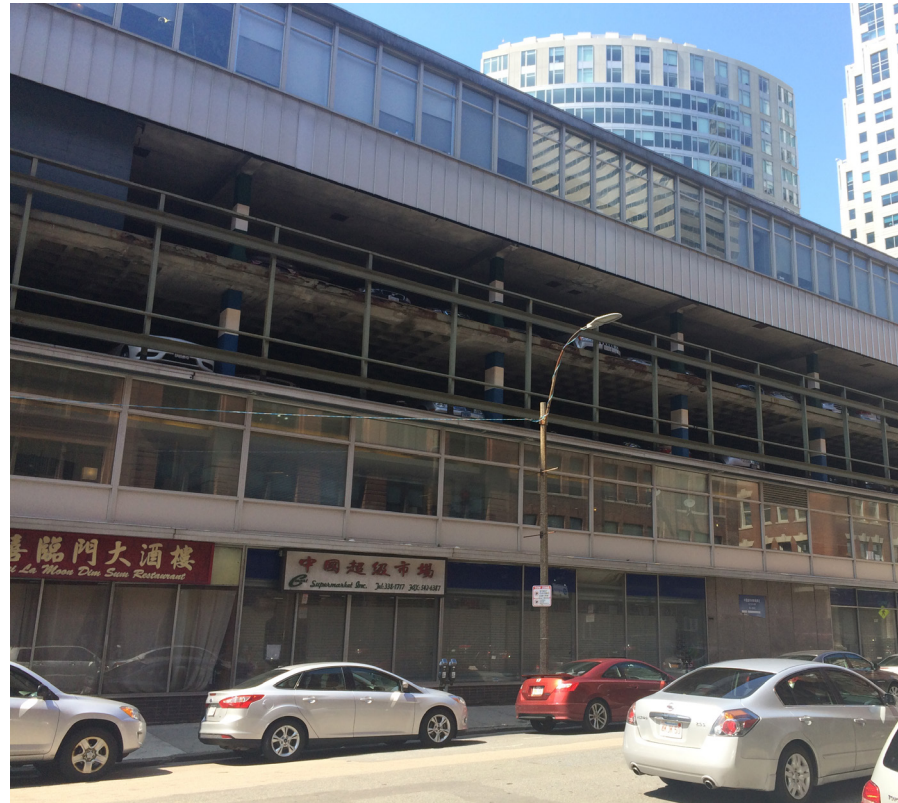
Lincoln St. Looking West
