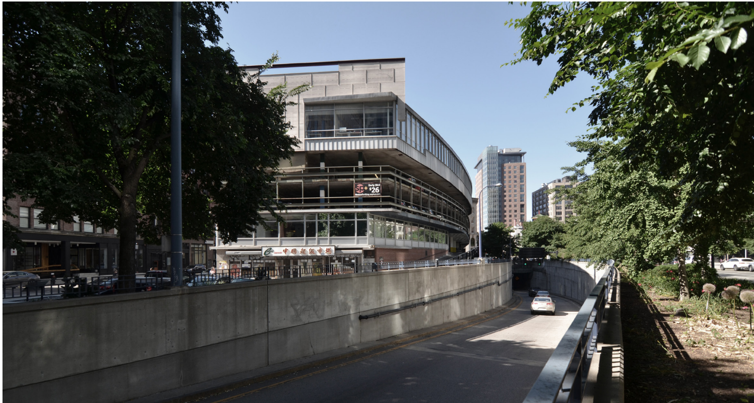
1-92 Ramp Looking South
