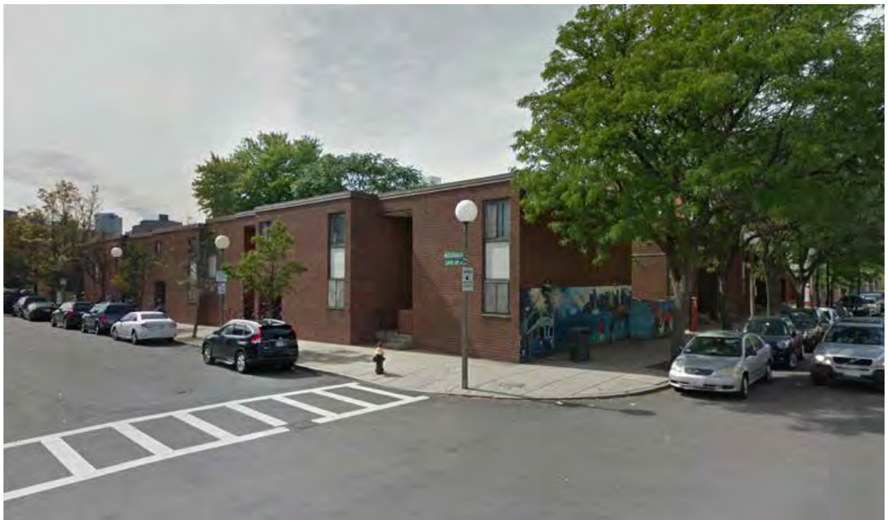
Photograph 2: View of the Site looking southwest from Sumner Street along Clipper Ship Lane
