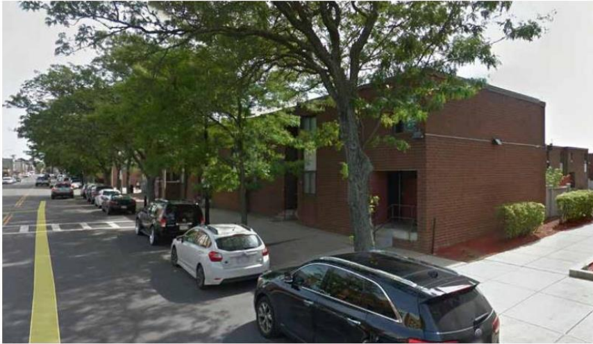
Photograph 1: View of the Site looking southeast along Sumner Street
