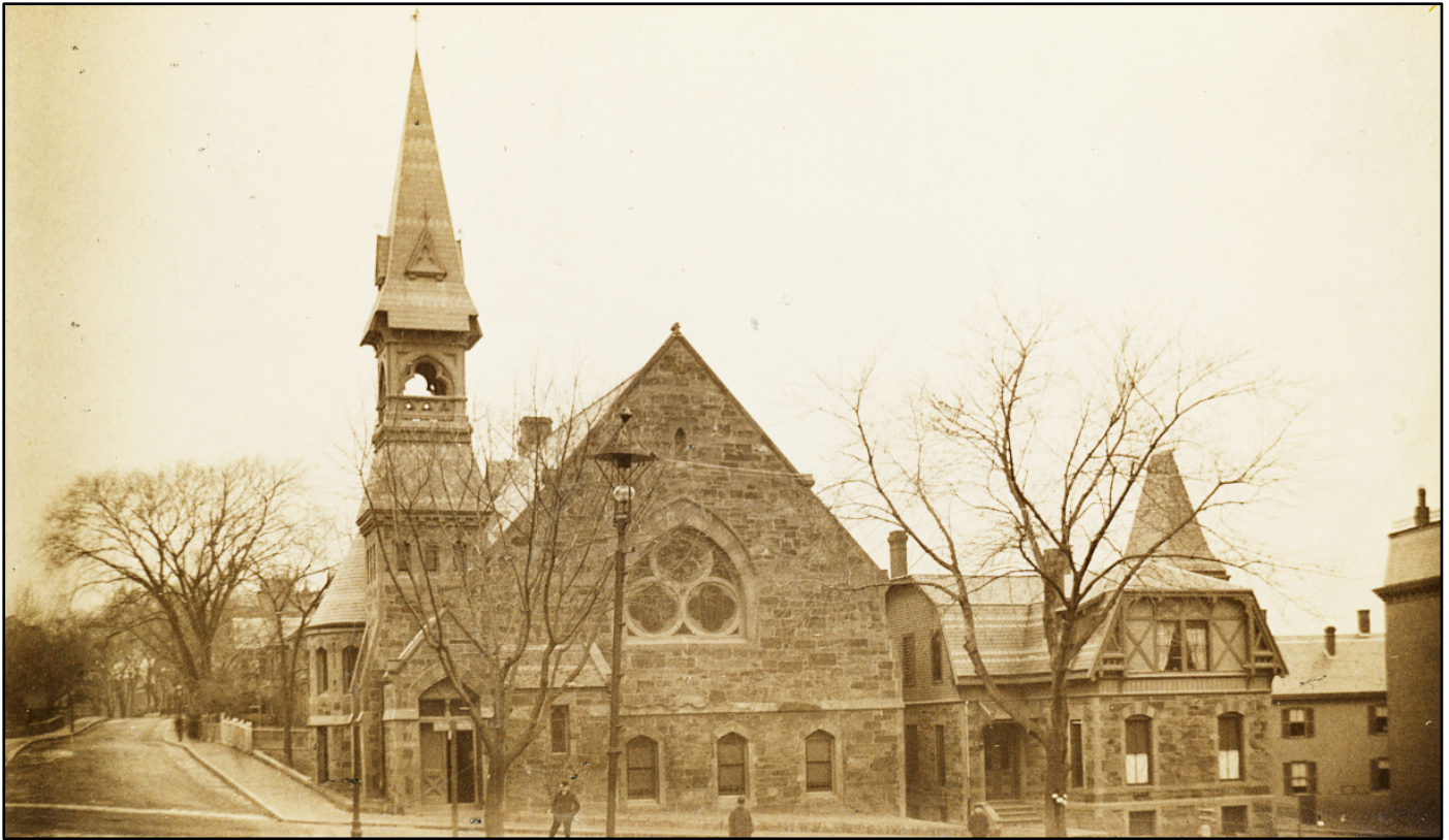
A view of the front façade of Church of the New Jerusalem at 3 Regent Street at Joseph Warren Square, at the corner of St. James Street in Roxbury, Massachusetts, built in 1874. A bell tower rises from the entranceway, behind which a turret stands on the St. James Street side of the church. On the façade, an arched window contains three quatrefoil round windows. This Swedenborgian church was established in 1870 and was later called the Roxbury Society of the New Jerusalem. The congregation disbanded in 1957, and the church was sold in 1958 and later occupied by the Church of God in Christ.
