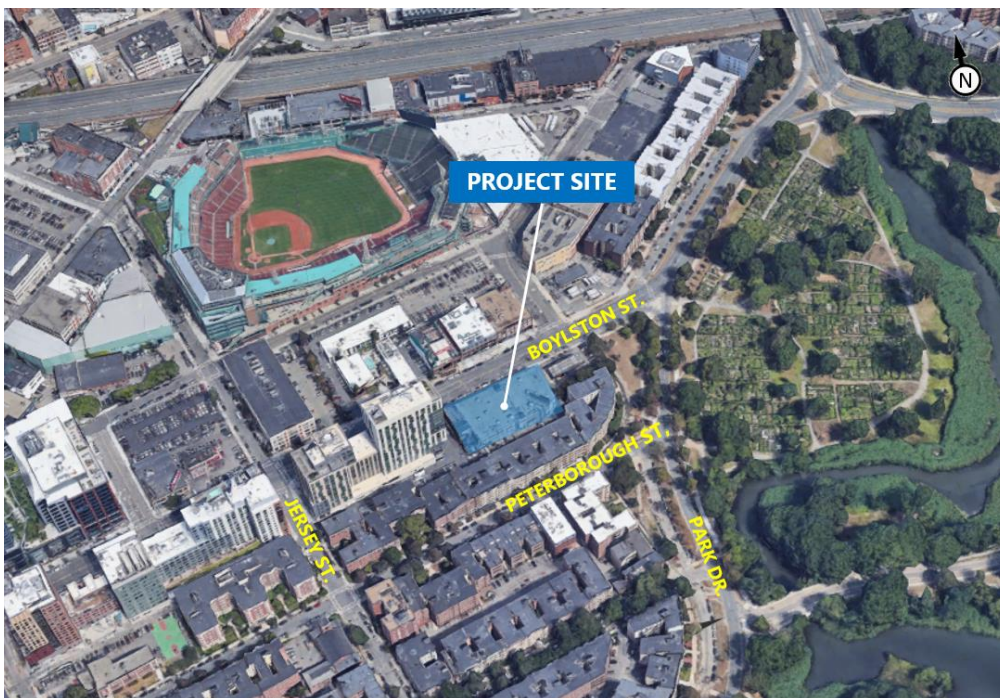
Image 1: Site Plan – Aerial View of the Existing Site and Surroundings (Courtesy of Google™ Earth)
