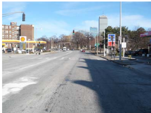
Figure 3-12 - Boylston Street looking eastbound
