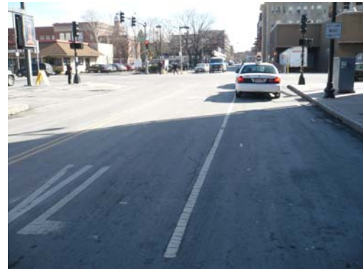
Figure 3-7 - Kilmarnock Street looking southbound
