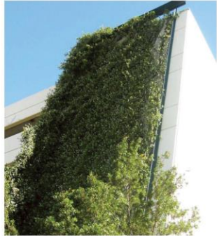
GREEN SCREENS ON PARKING GARAGE
