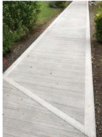
SAWCUT CONCRETE PATTERNS
