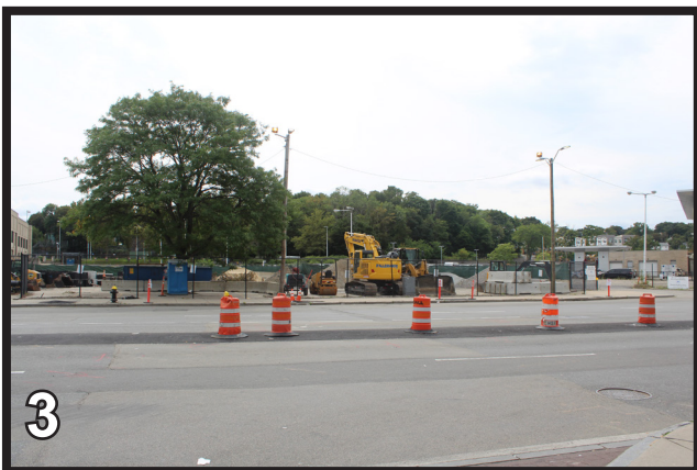
View of the Project Site from Dudley Square MBTA Station on Dudley Street
