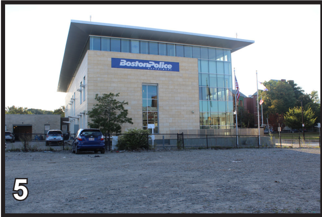
View of the Boston Police District B-2 Roxbury Station
