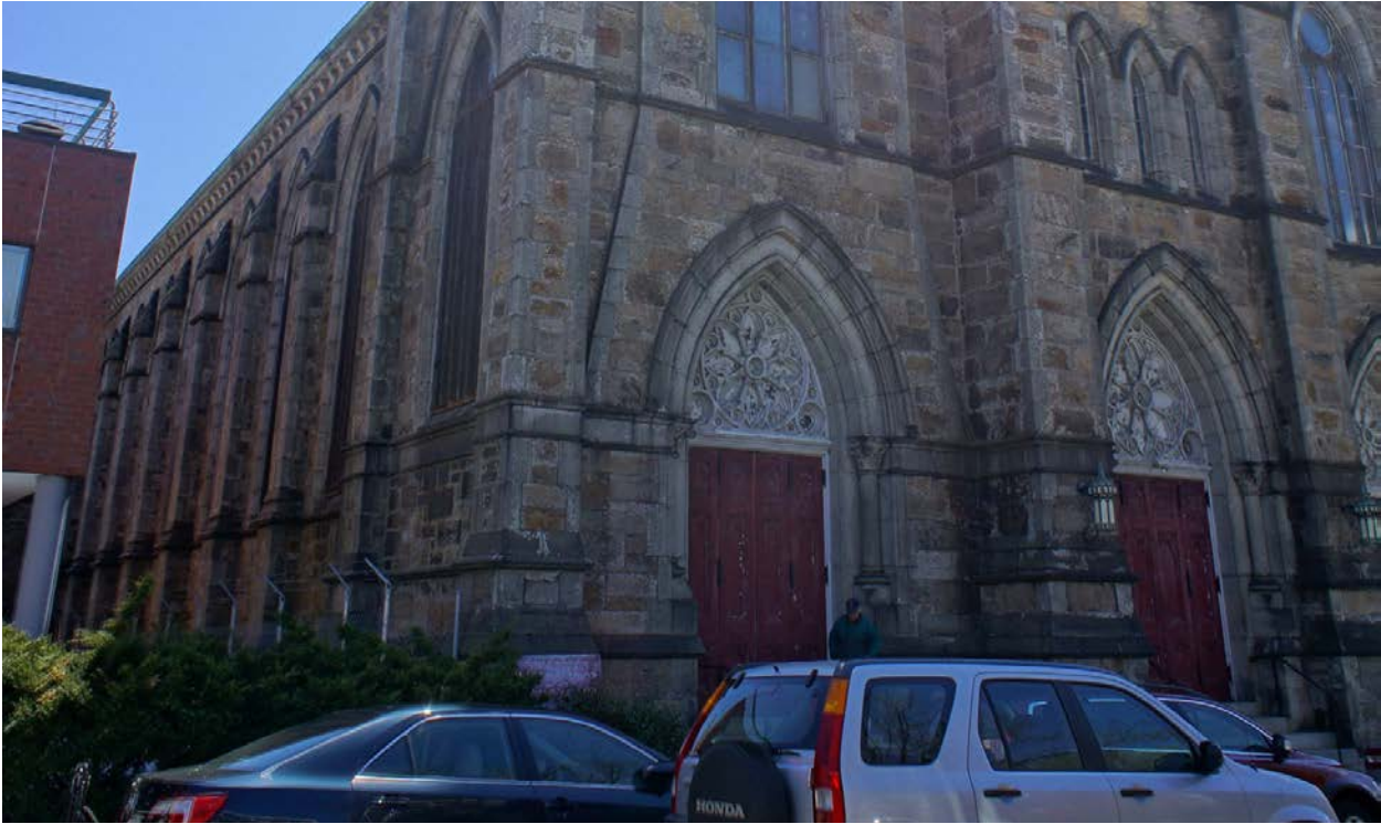
View Looking Southeast on Shawmut Avenue
