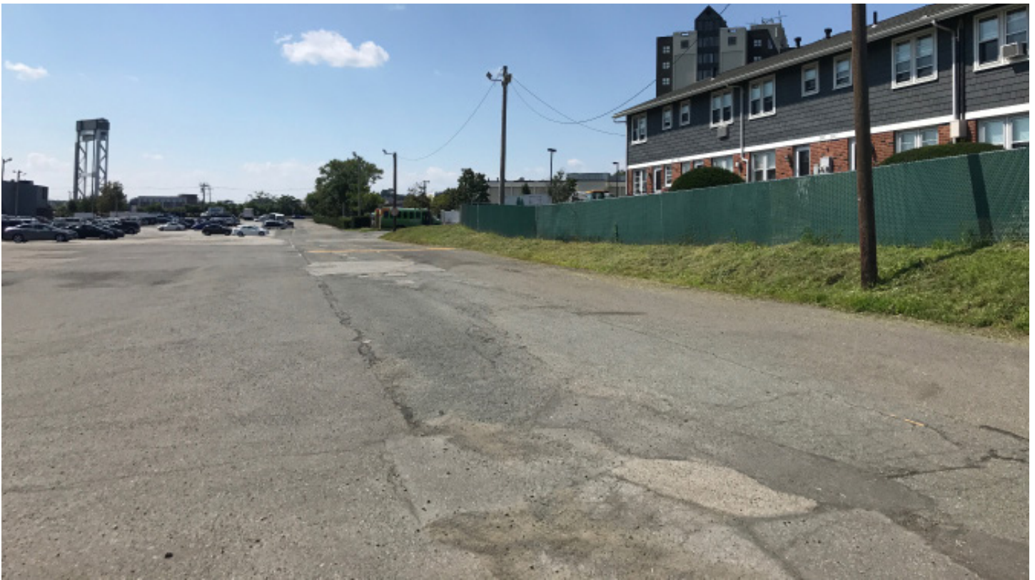
View 1: Project Site looking West - Brandywyne Village
