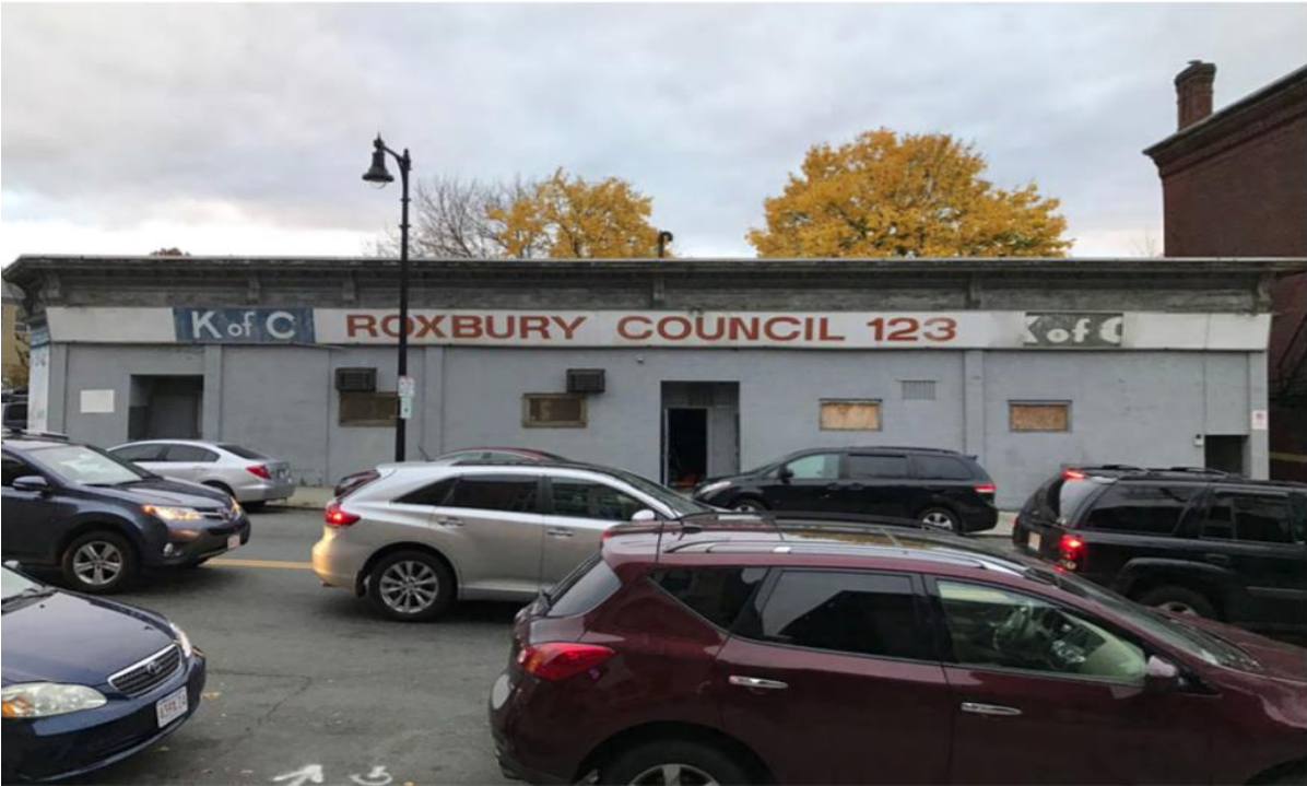
Photo 3 – Front on view of K&C site, facing north
