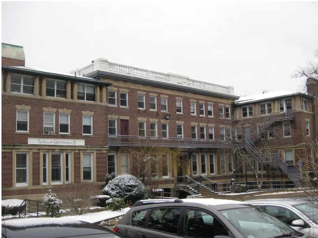
2. Home for Little Wanderers, 1914 Building (east elevation)
