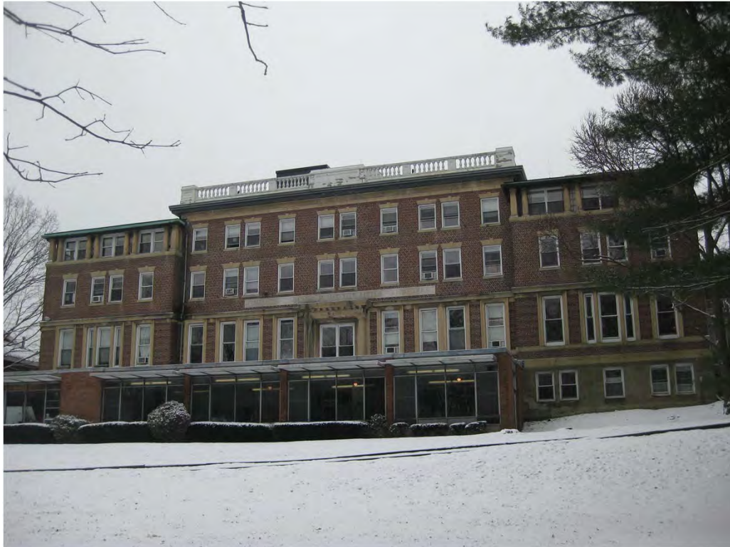
7 1914 Building and 1950s addition (west elevation)
