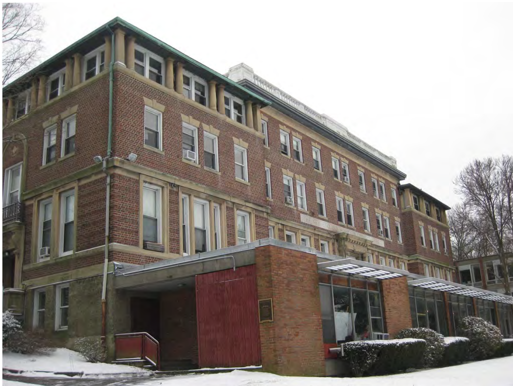
8. 1914 Building and 1950s addition (west elevation)
