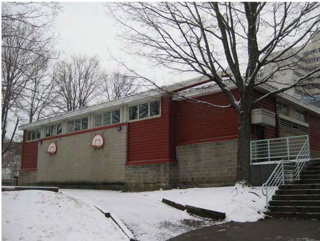
12. 1991 Gymnasium (west and south elevations)
