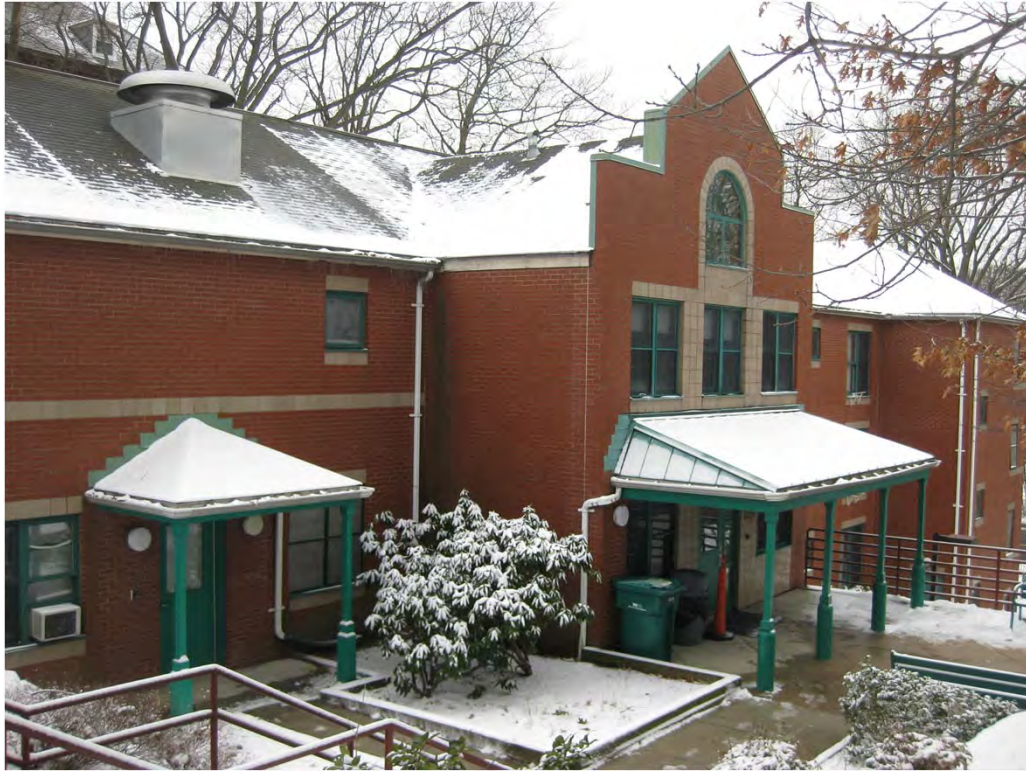
9. 1987 Residential Building (north elevation)
