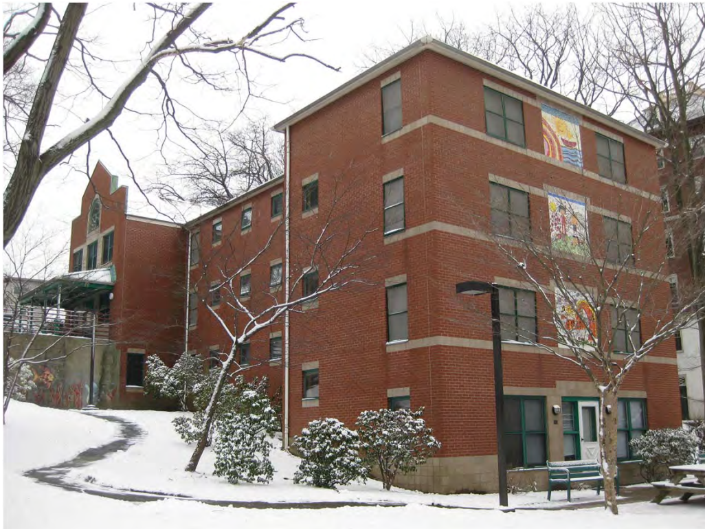
10. 1987 Residential Building (north and west elevations)
