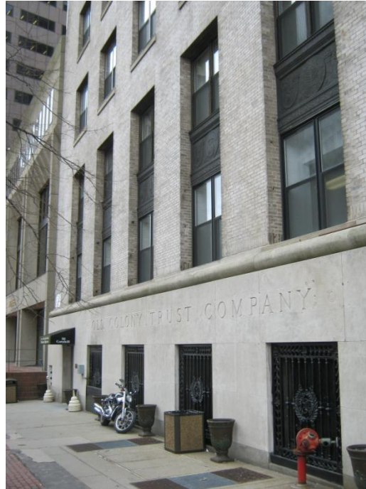
Figure 1-7: Cornhill St façade – Moakley Entrance
