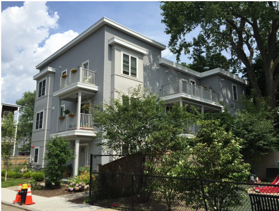
8 - 12 Stedman Street, Jamaica Plain ... 3-units, new construction
