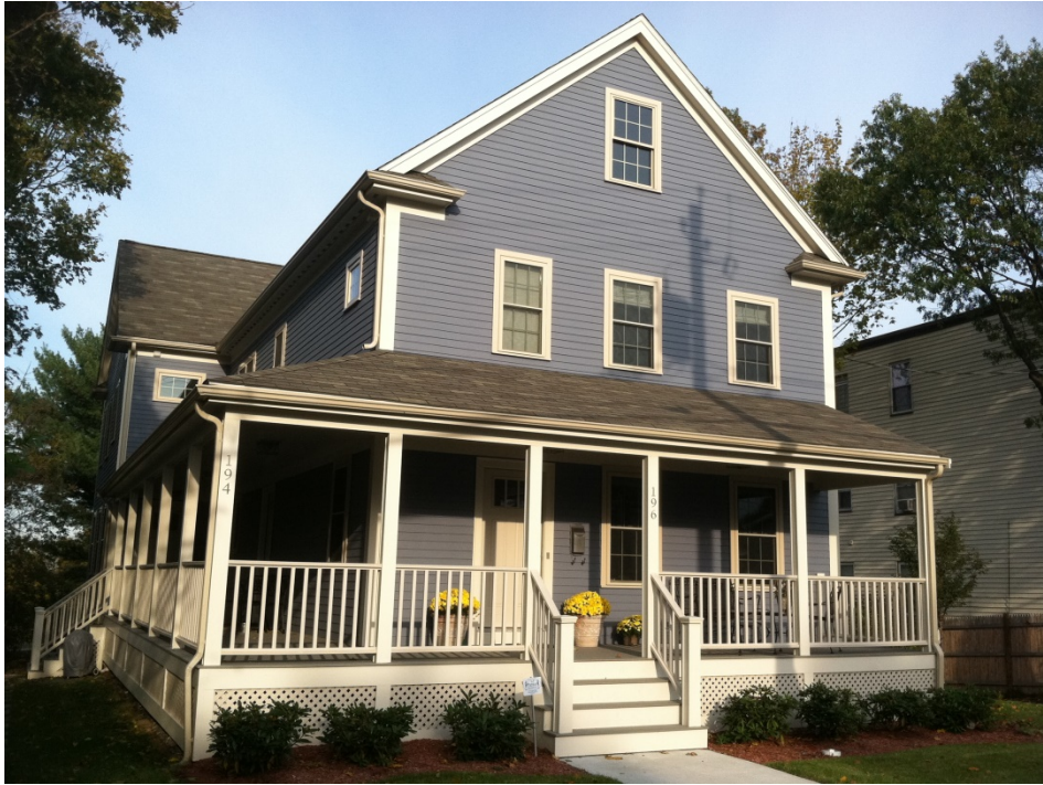
194 - 196 Durnell Avenue, Roslindale ... 2-units, new construction
