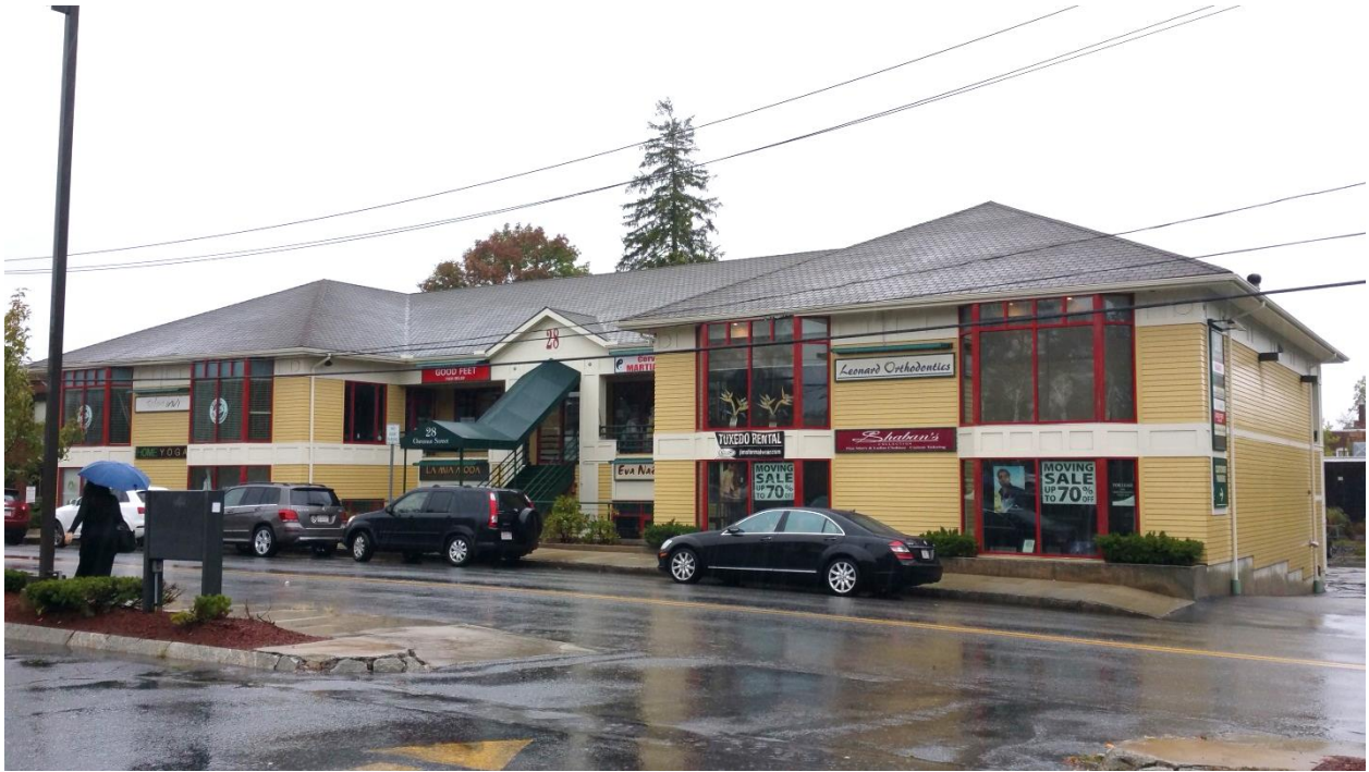
29 Chestnut Street, Andover, MA....commercial build-out, modernization
