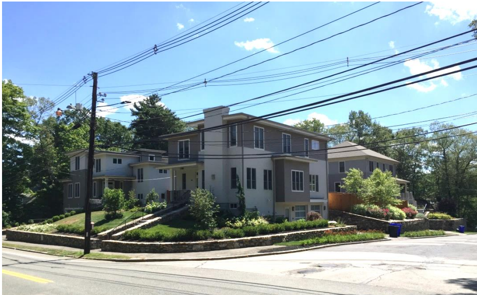
302 - 306 Allandale Road ... 3 single-families, new construction
