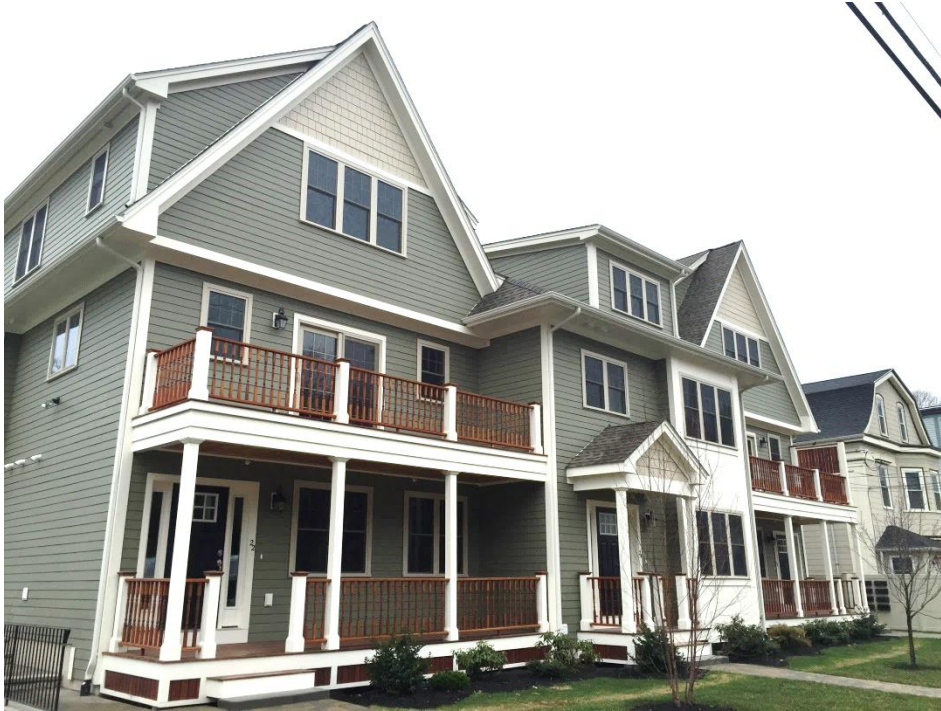
22 - 26 Hawthorne Street, Roxbury... 8-units, new construction
