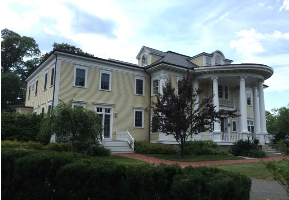
60 - 64 Pond Street, Jamaica Plain ... 3-unit conversion, restoration
