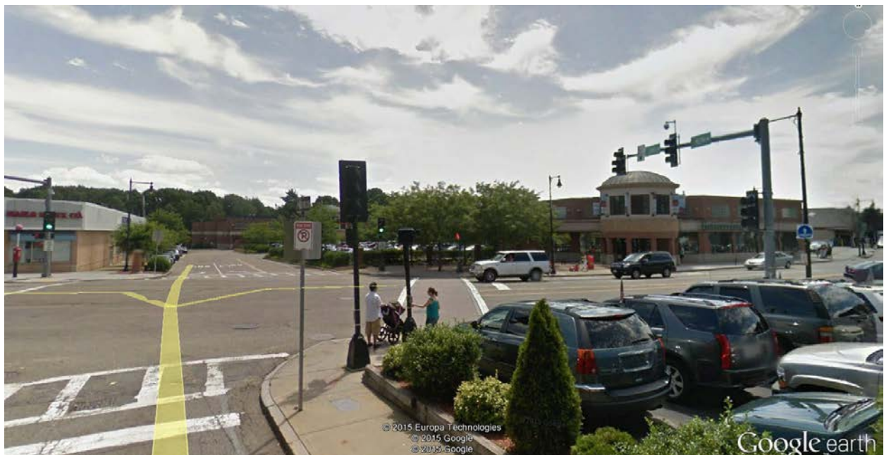
View of proposed project site looking south on Willow St. towards the entrance to Roche Bros.
