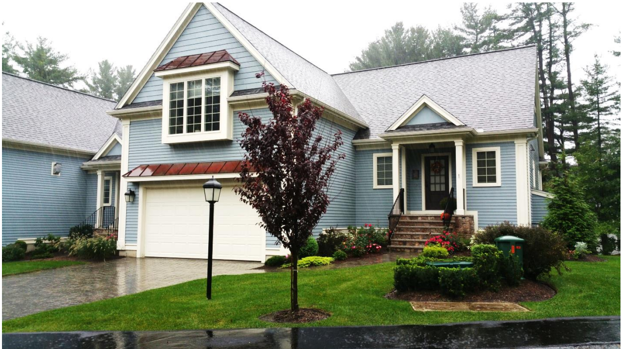
Lincoln Woods, Andover, MA....24-Residential townhouse units, new construction
