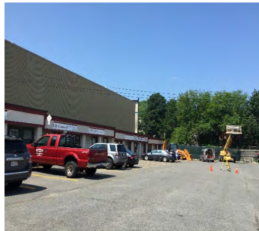
VIEW OF EXISTING BUILDING FROM INSIDE LOT
