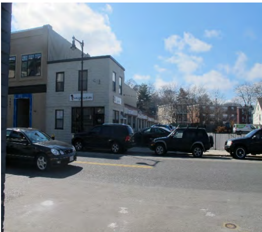
VIEW OF EXISTING BUILDING ON SITE
