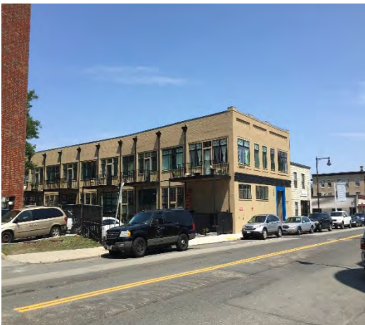
VIEW OF RESIDENTIAL BUILDING ADJACENT AT 1861, PEABODY SQUARE LOFTS
