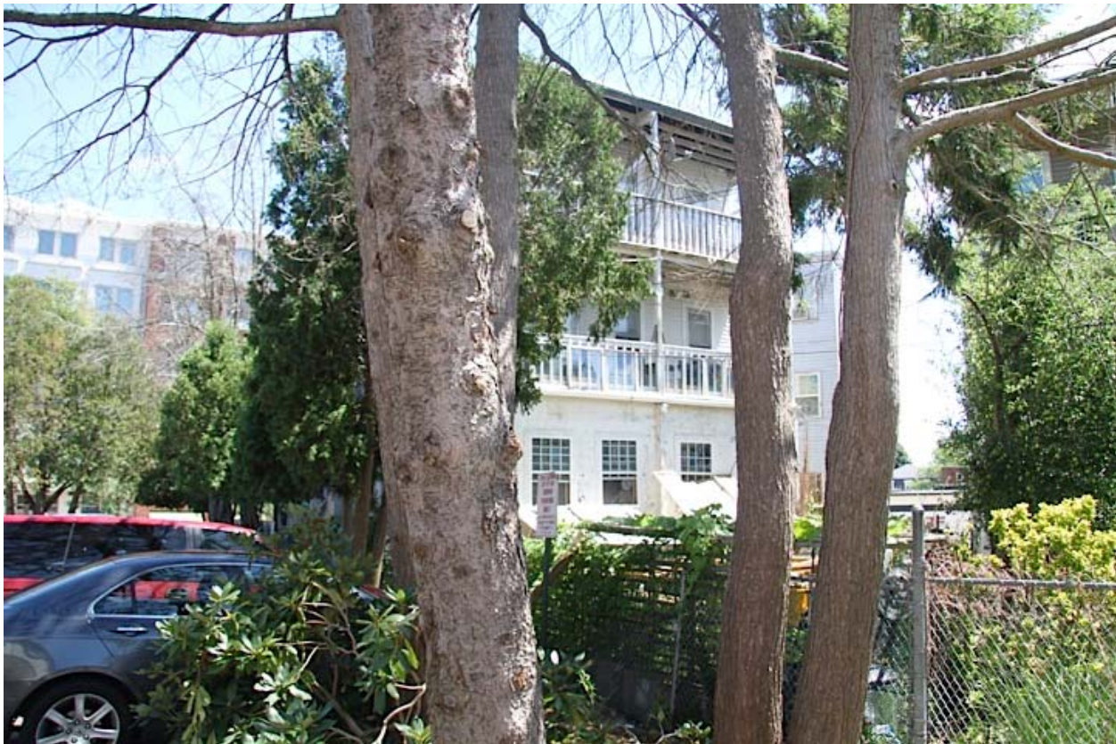
View D -- Adjacent triple-decker (existing) on Dorchester Avenue
