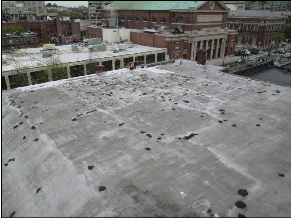
9. Main theater roof – built-up roof
