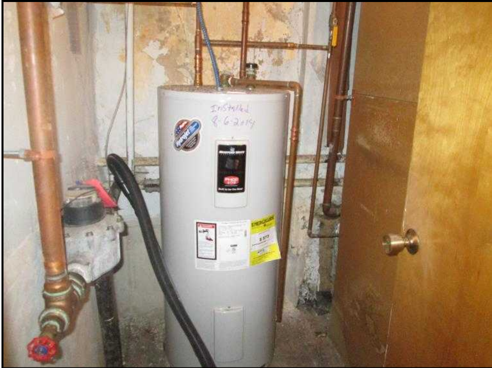
29. 252 Huntington electric water heater
