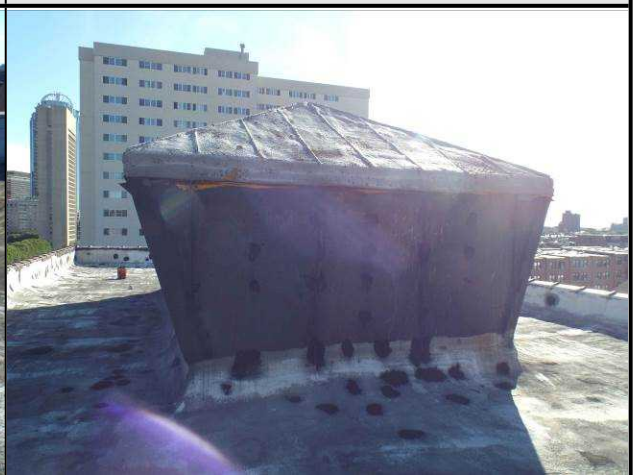
High roof over stage with ventilator
