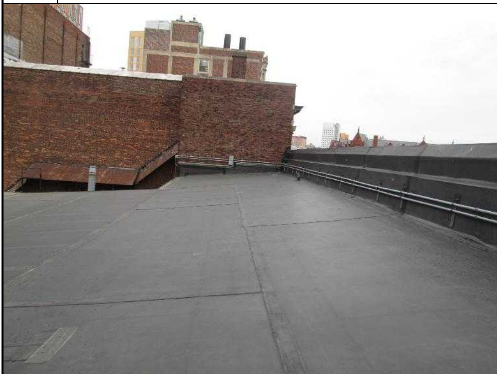
18. 258 Huntington roof – EPDM roof
