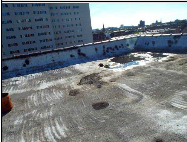
High roof over stage
