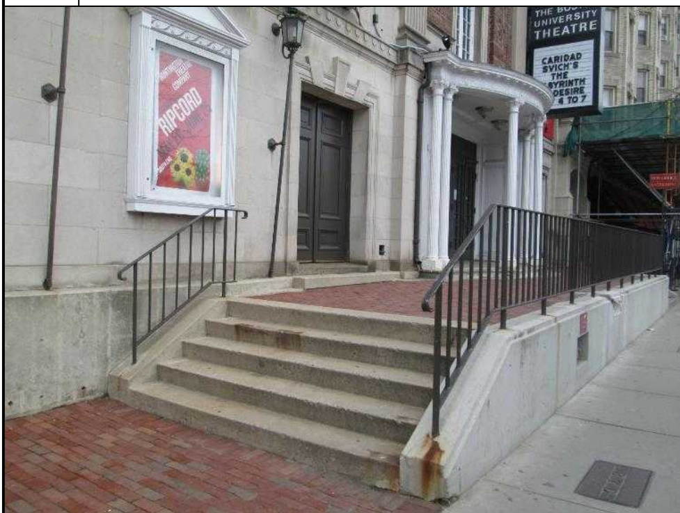
8. Exterior concrete stairs
