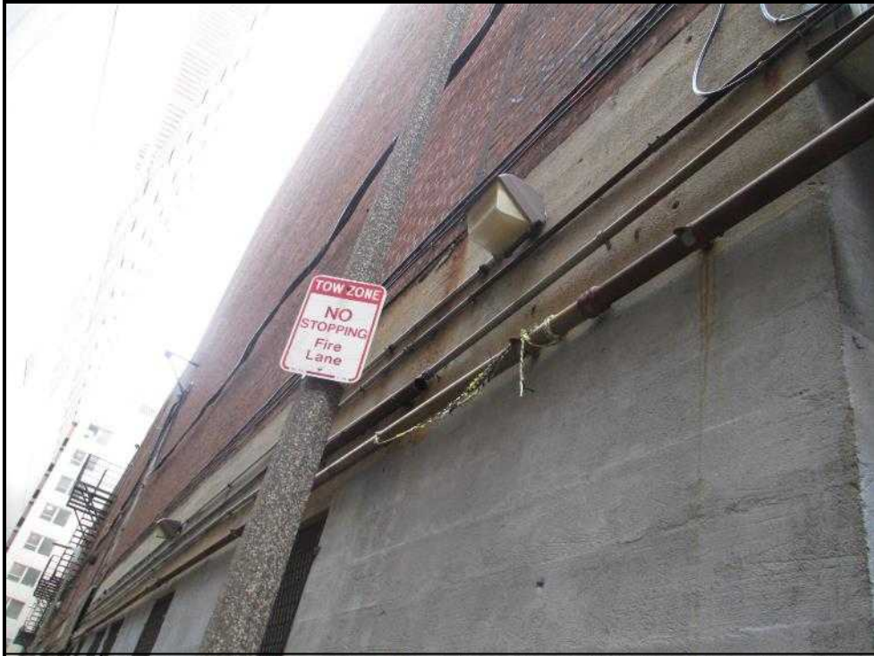
5. Rear façade of building
