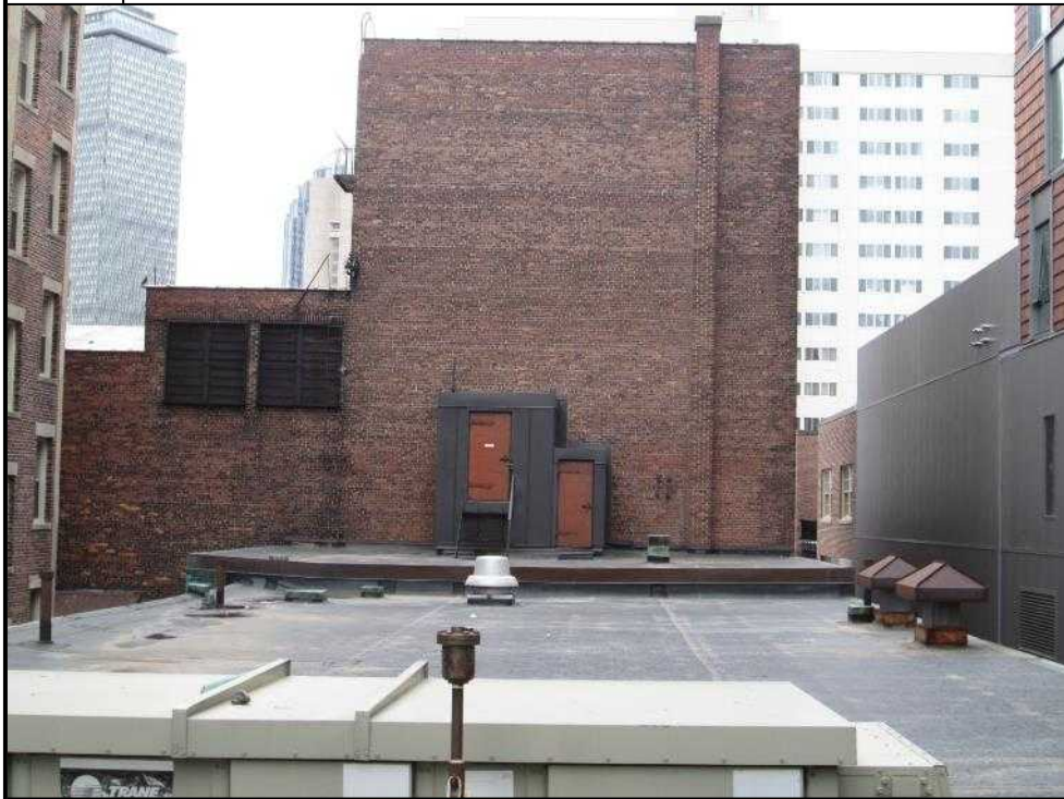
4. South façade of building
