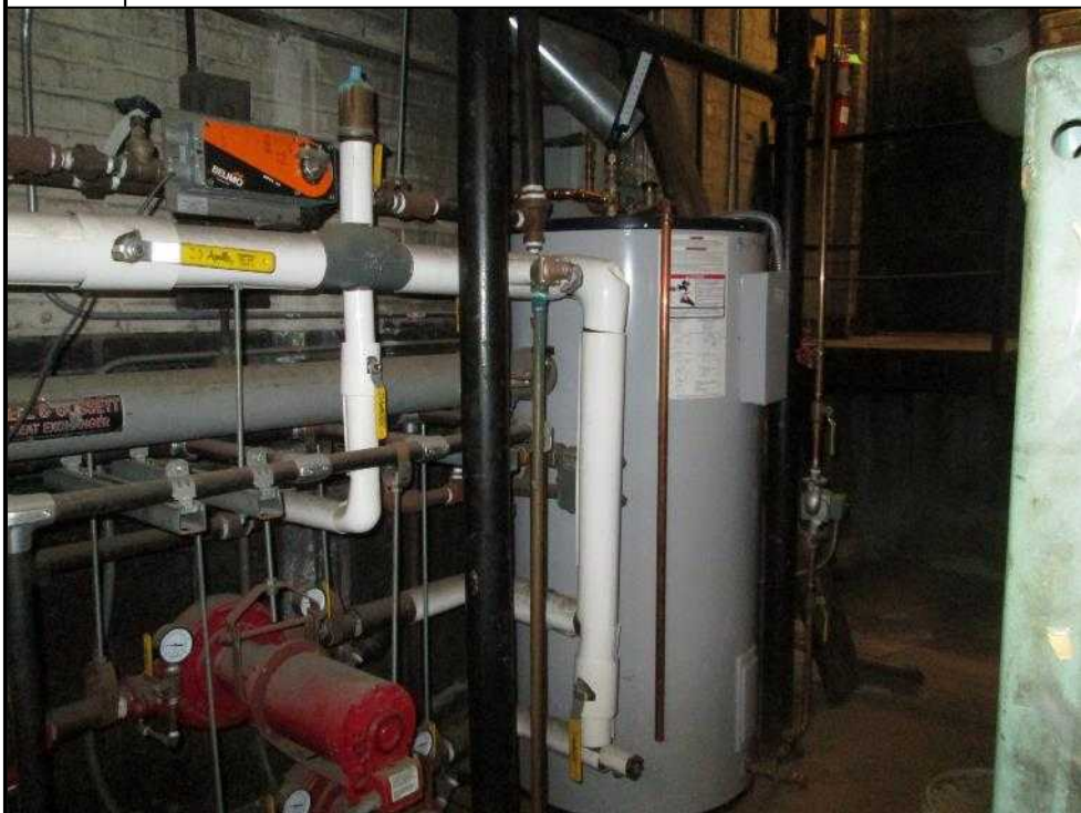
28. Electric water heater
