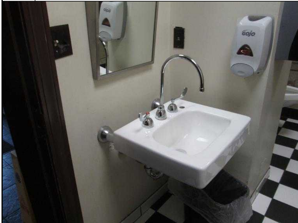
20. Public bathroom finishes and fixtures
