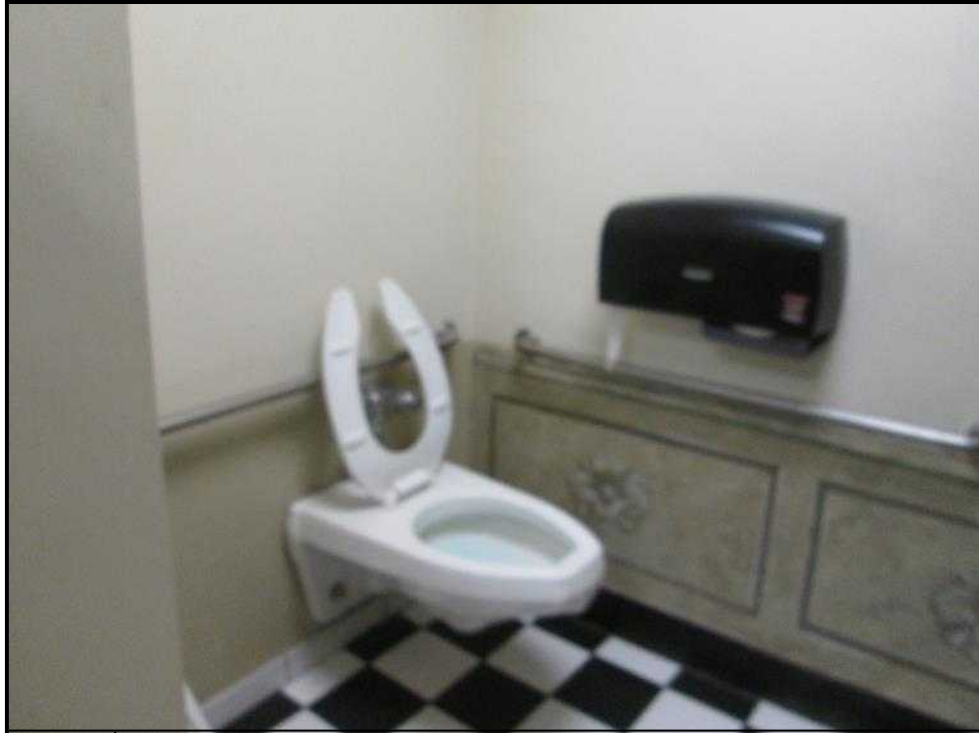
19. Public bathroom finishes and fixtures
