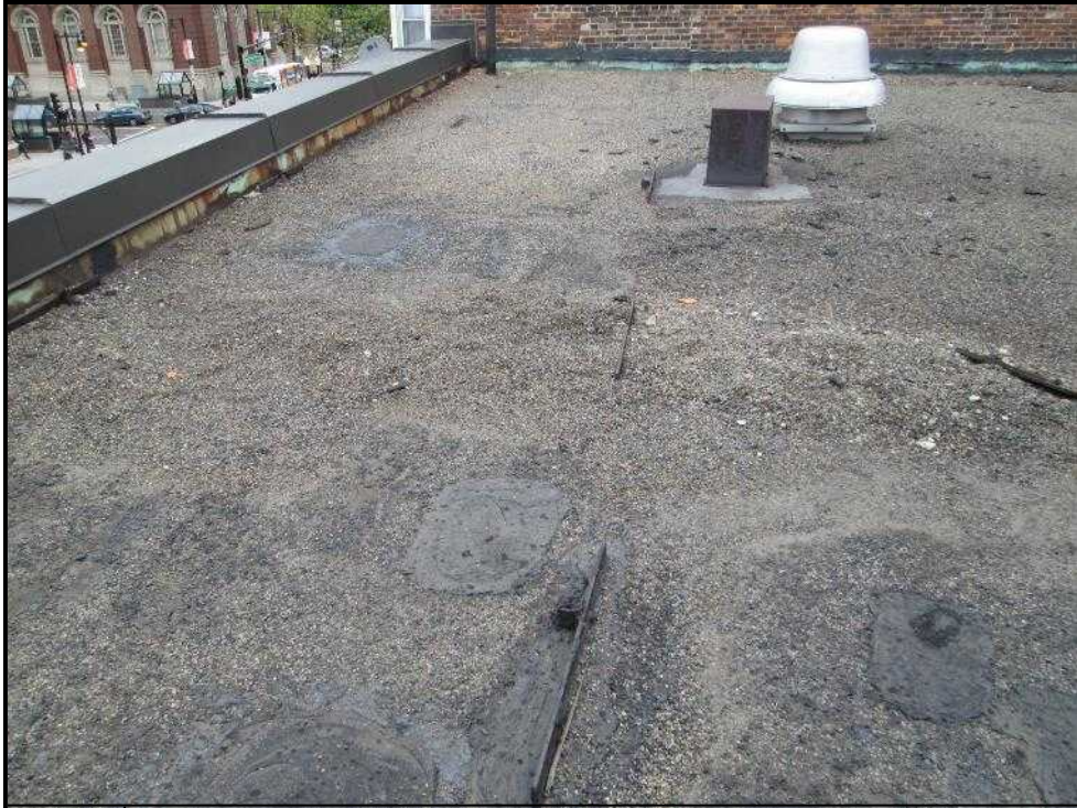
11. 252 Huntington roof – built-up roof
