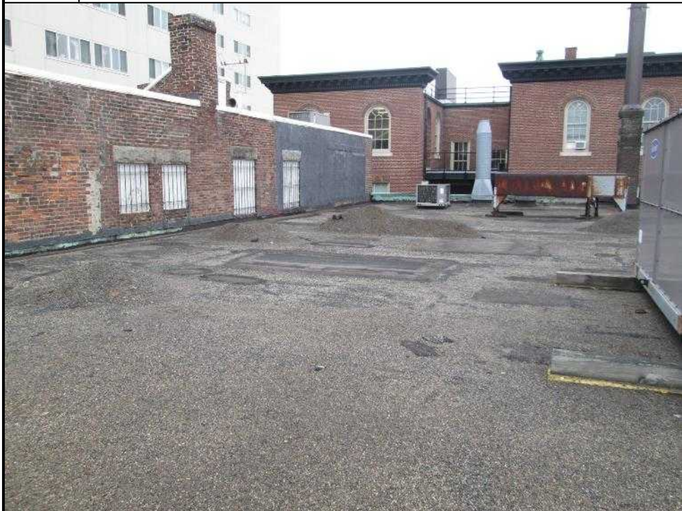
10. 252 Huntington roof – built-up roof
