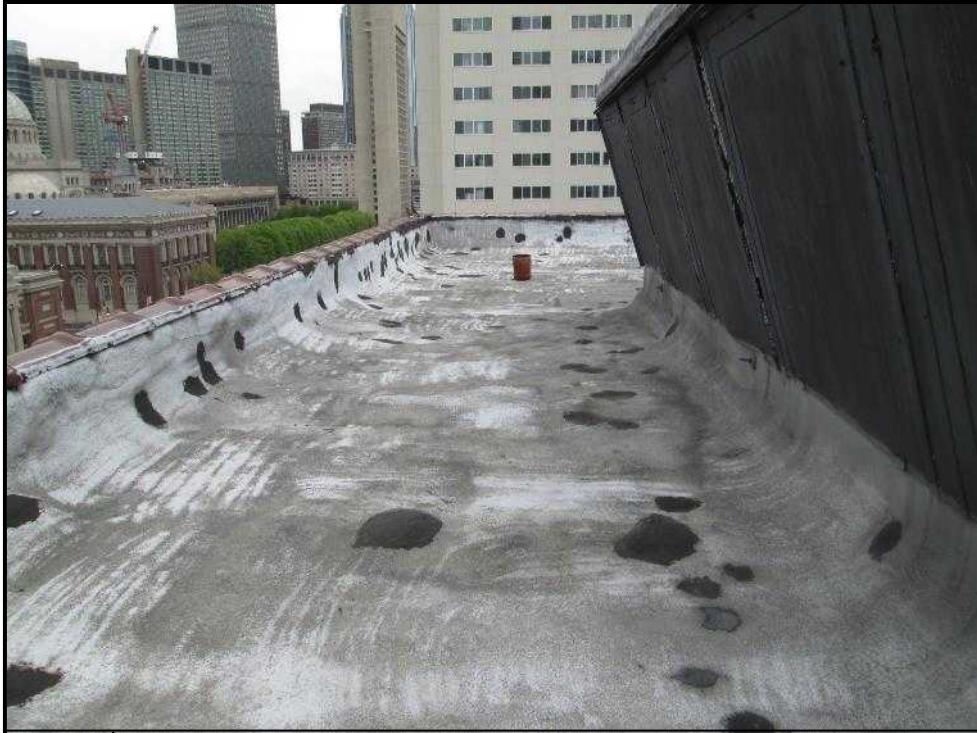
11. Main theater roof – built-up roof
