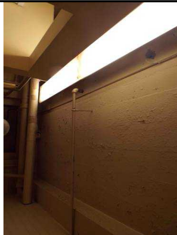
Finishes in basement
