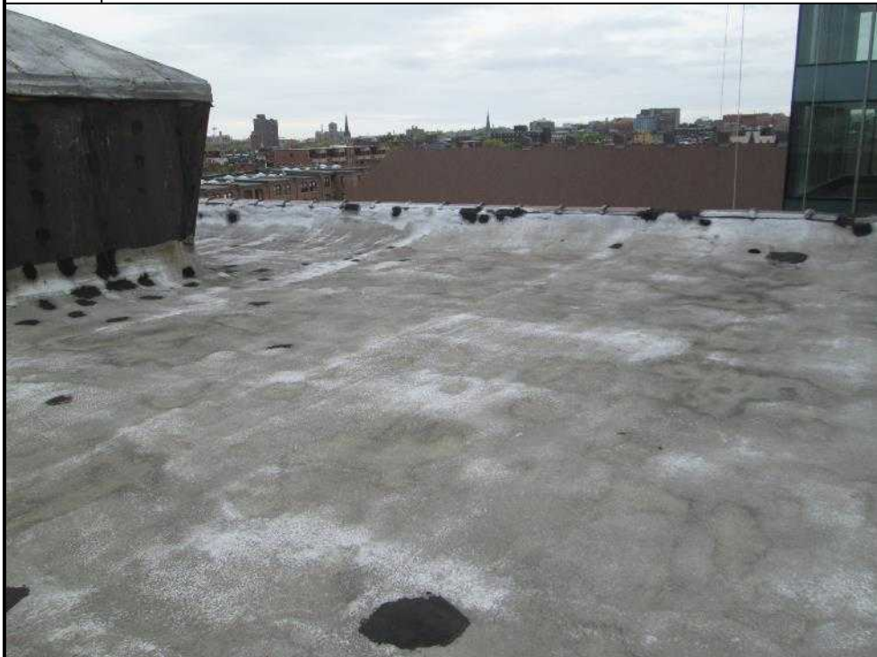
10. Main theater roof – built-up roof
