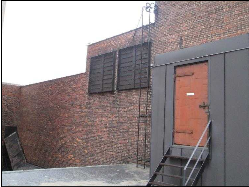
3. South façade of building
