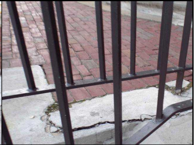
Spalled concrete
