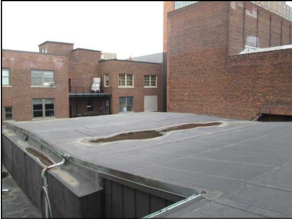
17. 258 Huntington roof – EPDM roof
