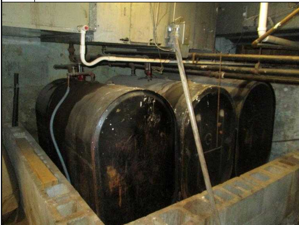
28. 252 Huntington oil tanks
