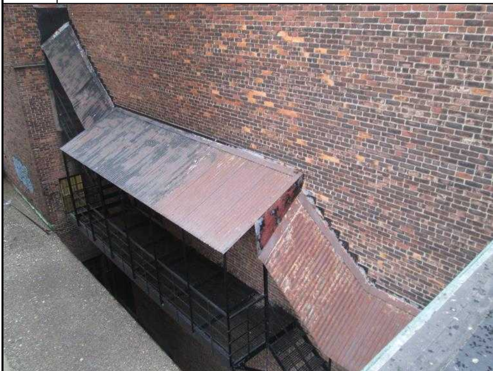
6. Exterior fire escape stairways
