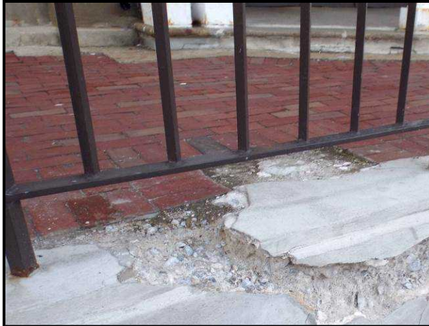
Spalled concrete
