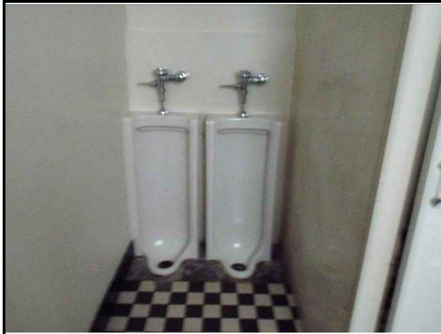
Typical bathroom in "L"
