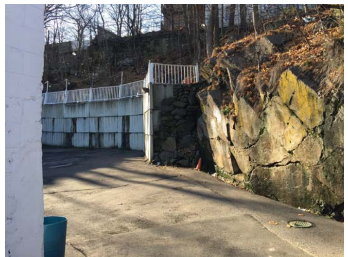
Back Lot Retaining Wall
