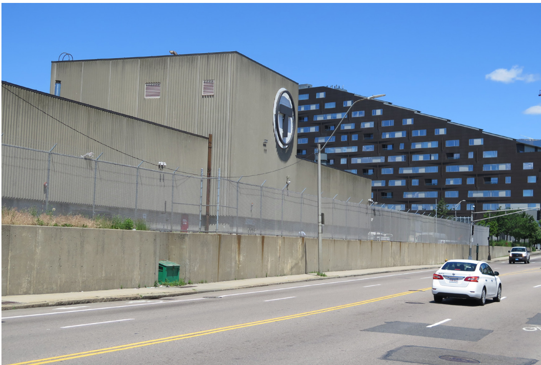
Nearby MBTA Storage Yards on Dorchester Avenue
