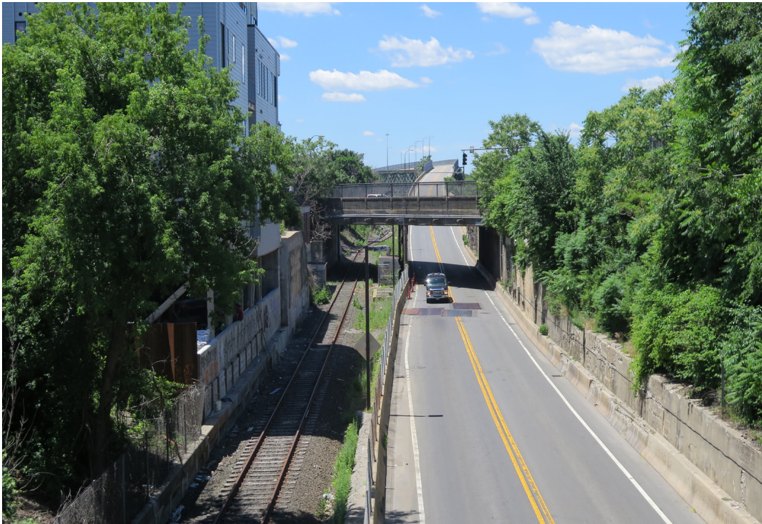
Adjacent Haul Road
