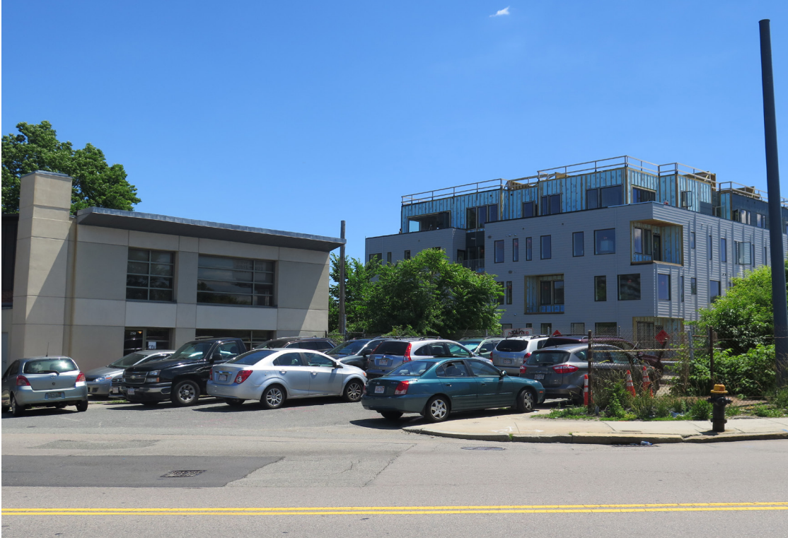
Parking on Private Street next to Existing Building and Adjacent Residential Structure (under construction) on otherside of the Haul Road
