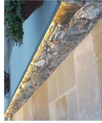
Stone Veneer Retaining Wall with LED Strip Lighting
