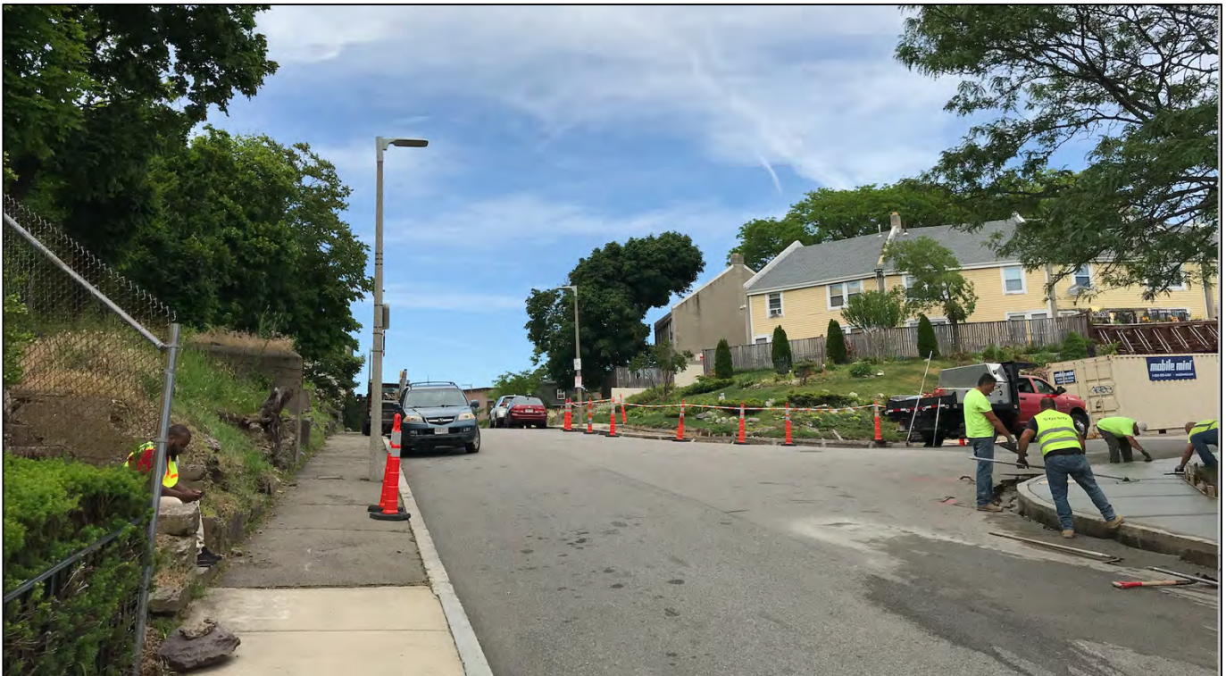
View of Sidewalk Immediately Adjacent to 25 Fountain
