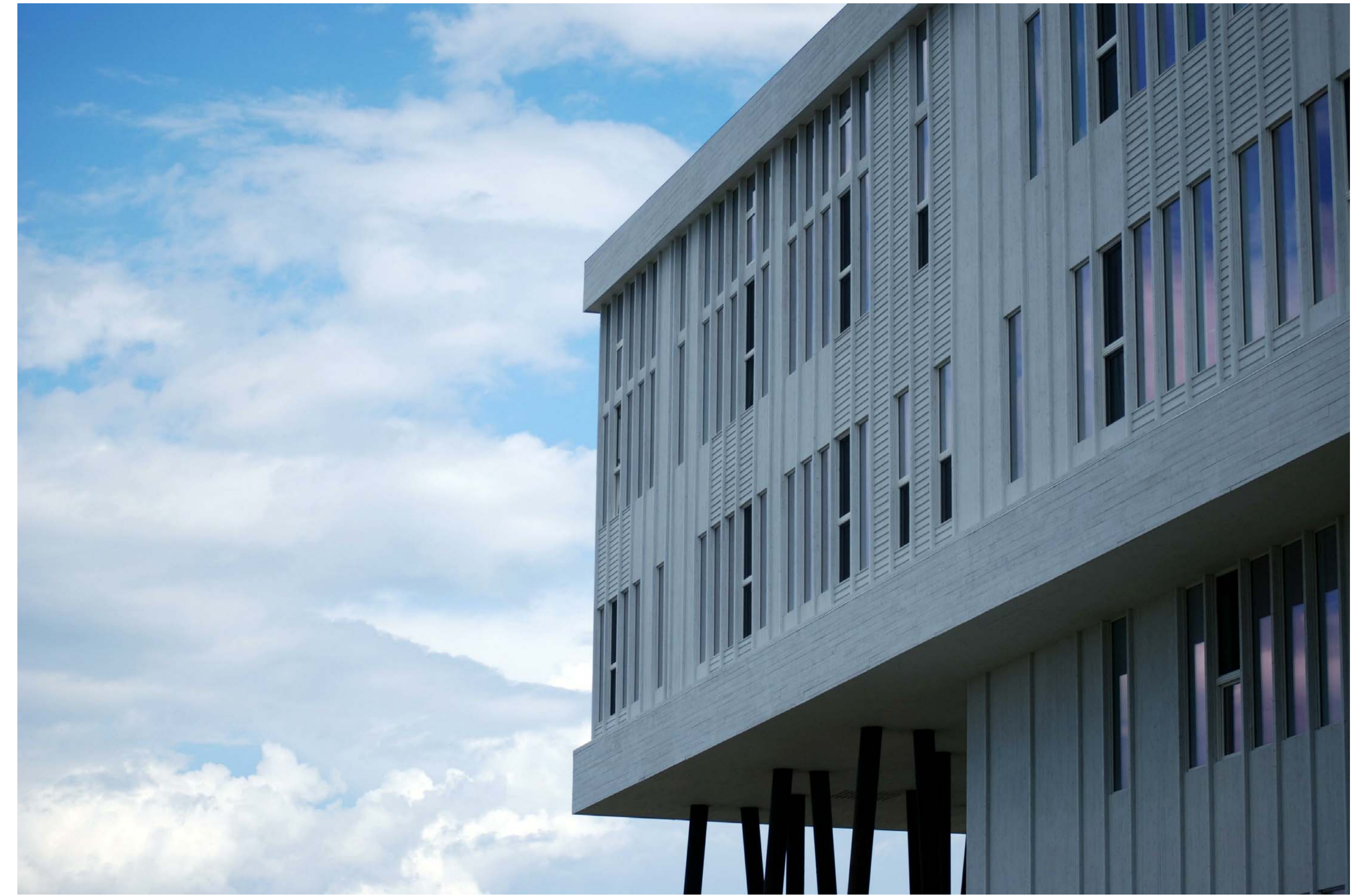
VARIED WOOD SHIPLAP FOGO ISLAND INN, NEWFOUNDLAND SAUNDERS ARCHITECTURE
