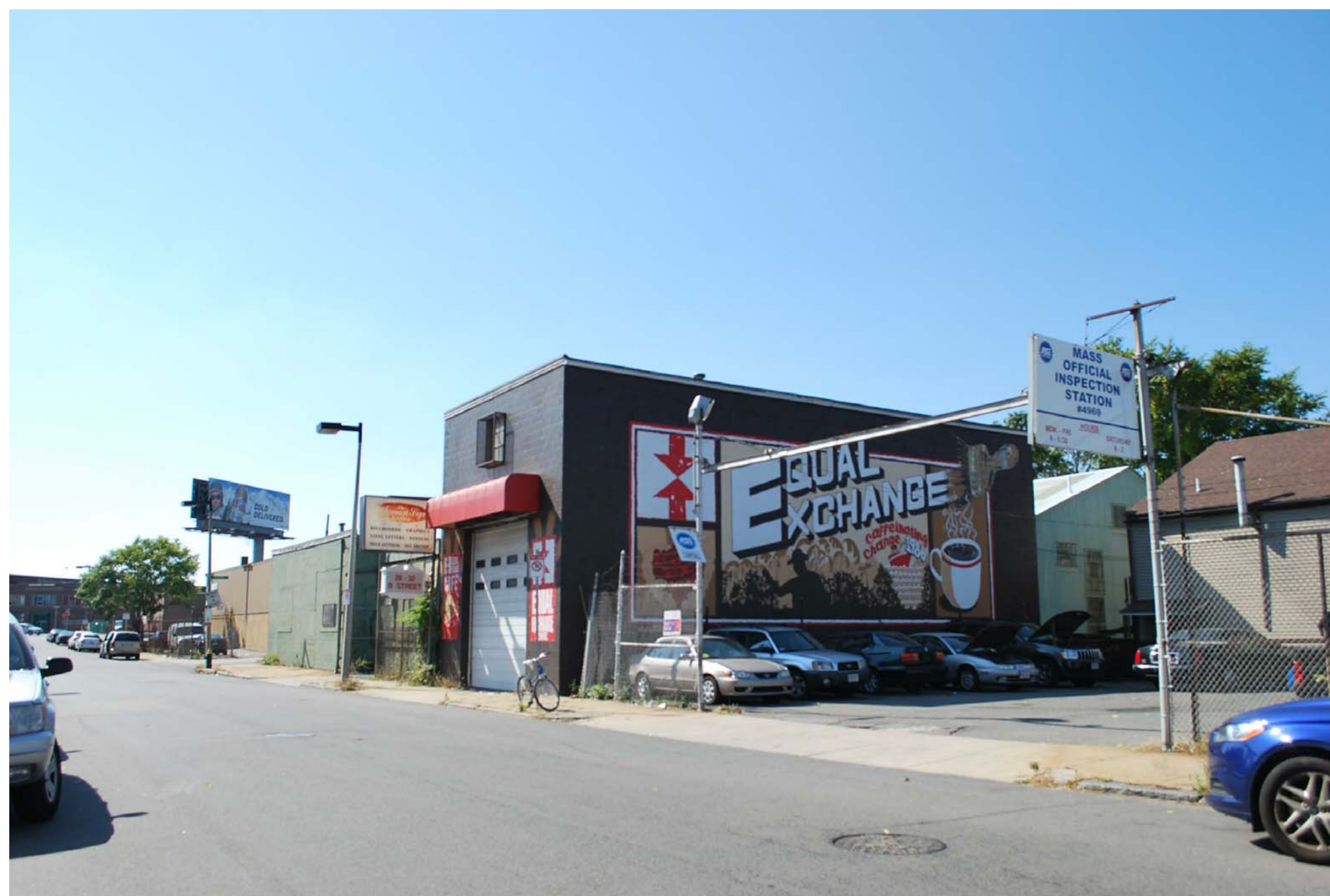
EAST CORNER OF SITE
