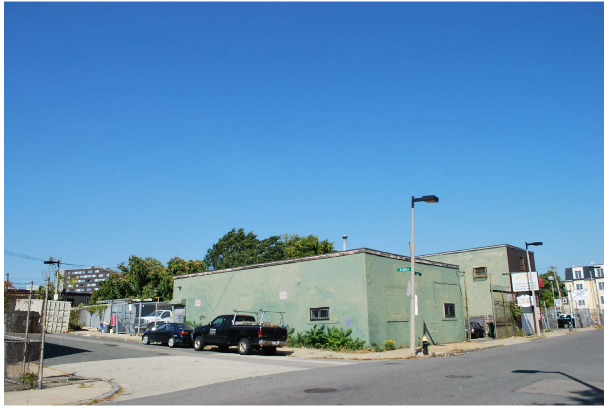
SOUTH CORNER OF SITE
