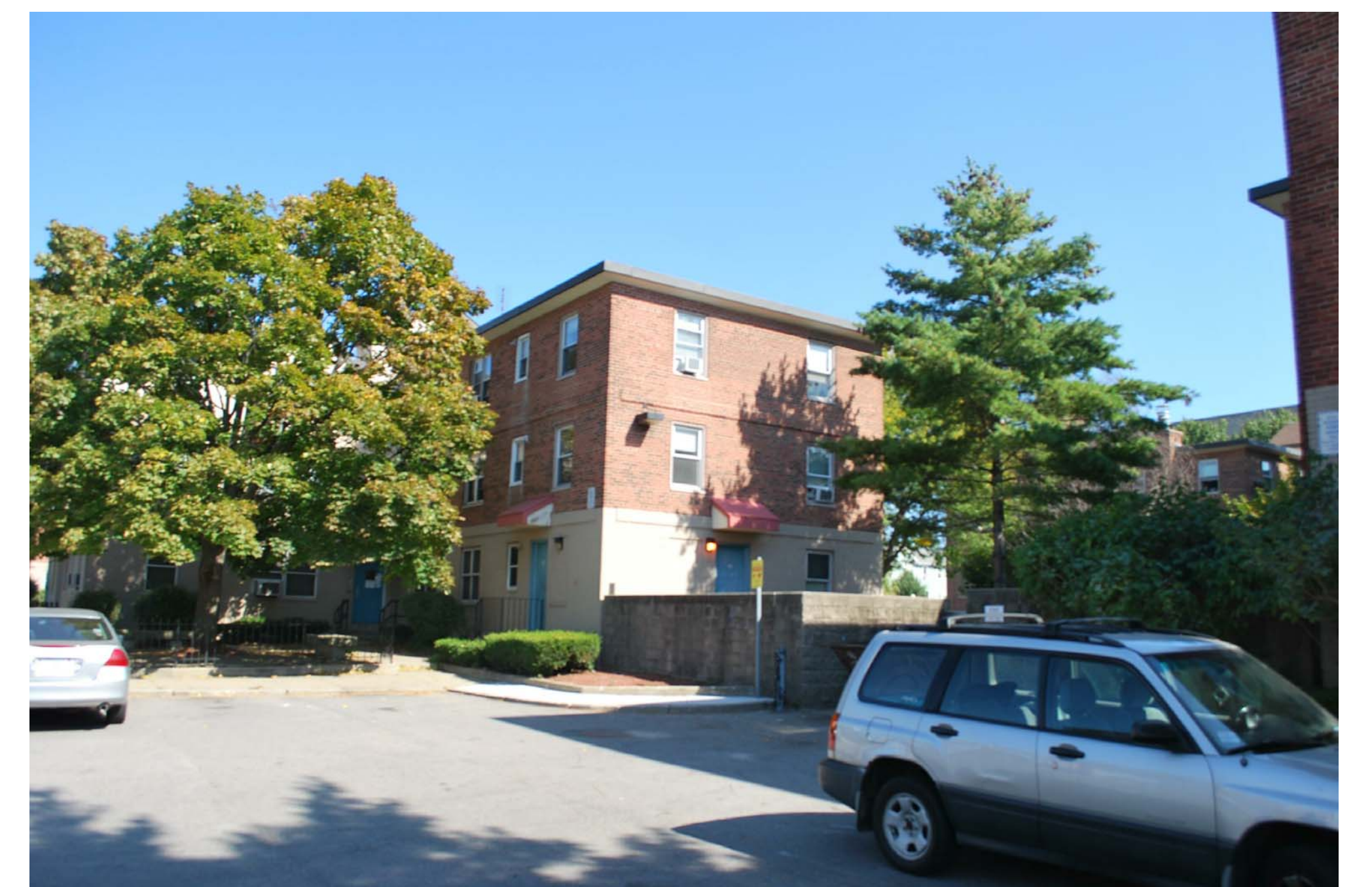
3 STORY HOUSING ACROSS 'B' STREET
